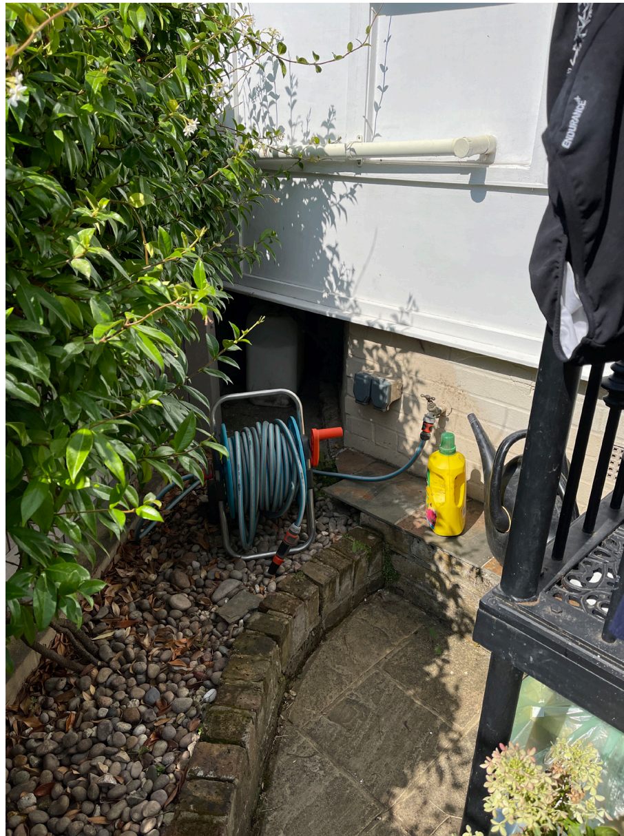
The conservatory has been raised to create level access to the existing apartment.
