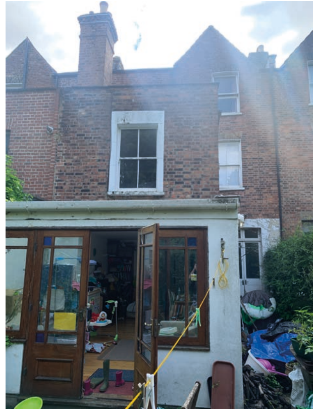
3. Existing rear facade with lean-to extension and side access from the kitchen.
