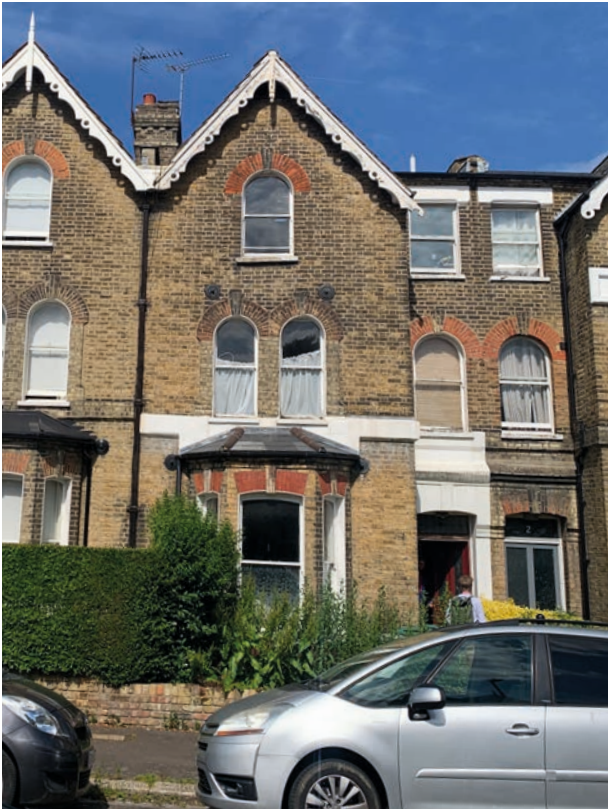
2. Existing front facade showing the architectural expression of the terrace and the neighbouring properties
