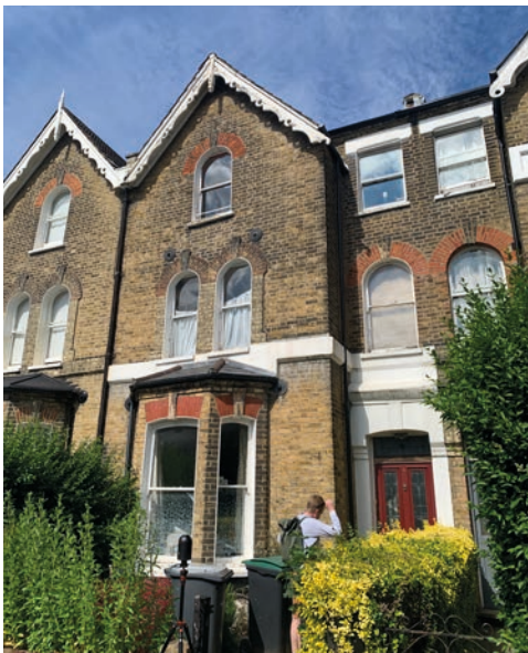
Bins are currently kept in the front garden, no dedicated storage space is currently provided.
