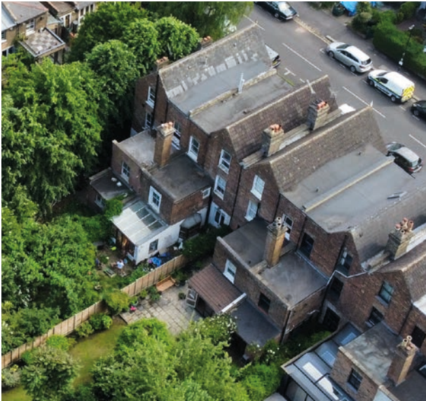
1. Aerial photo to the rear of the application site.
