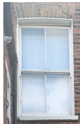
Existing Rear Windows
