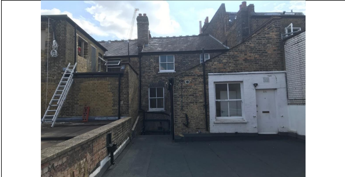
Plate 1: Photograph of the rear elevation and outrigger from above the single-storey element
