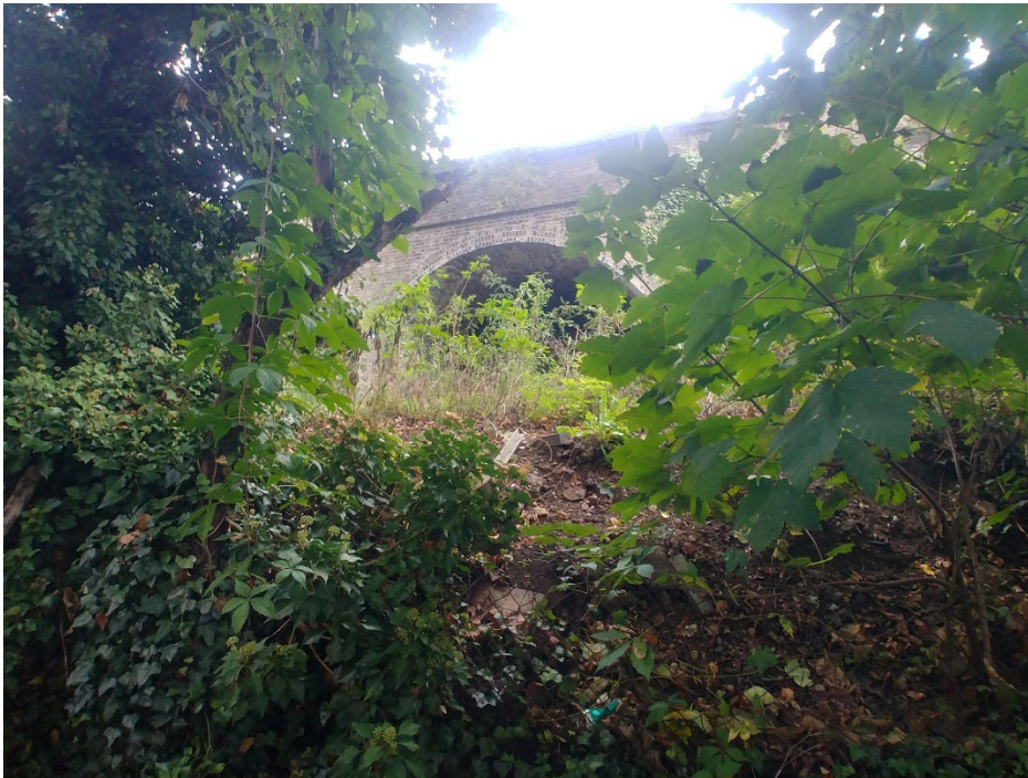
Plate 4 – Railway arches as viewed from the north east boundary of the Grace Centre.
