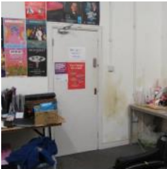
Figure 3: Existing post room
