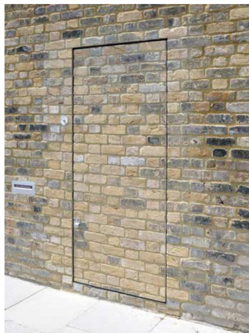
Brick Slip Doorway
