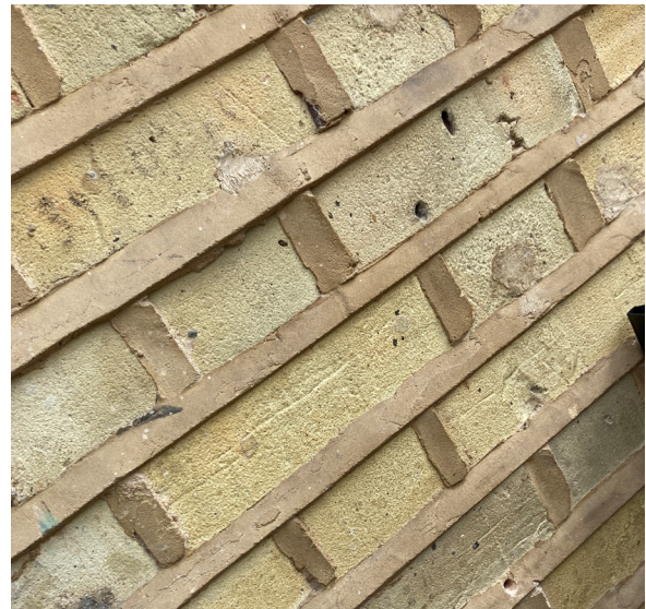
Figure 2: Existing brickwork pointing behind visitor services desk
