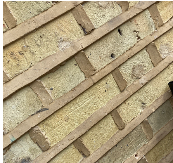
Figure 2: Existing brickwork pointing
