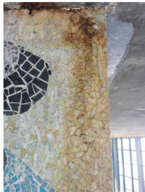
Images 6a-b – Staining caused by rust and saline efflorescences
