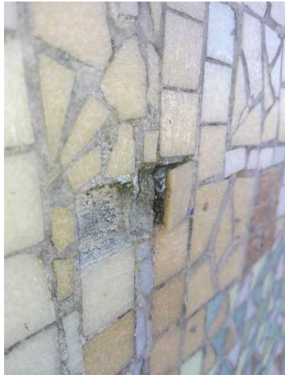
Images 4a-b – Detachment of tesserae from the substrate
