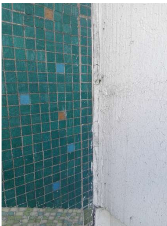
Image 10 – Stainless steel strip along vertical side ends
