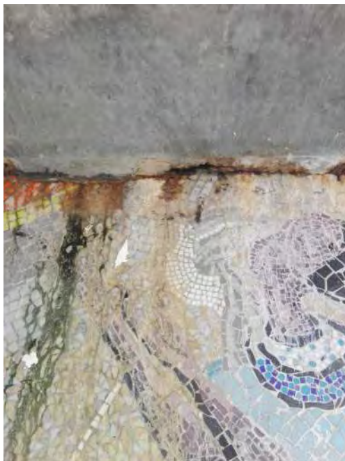
Images 6a-b – Staining caused by rust and saline efflorescences
