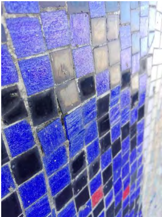
Images 4a-b – Detachment of tesserae from the substrate
