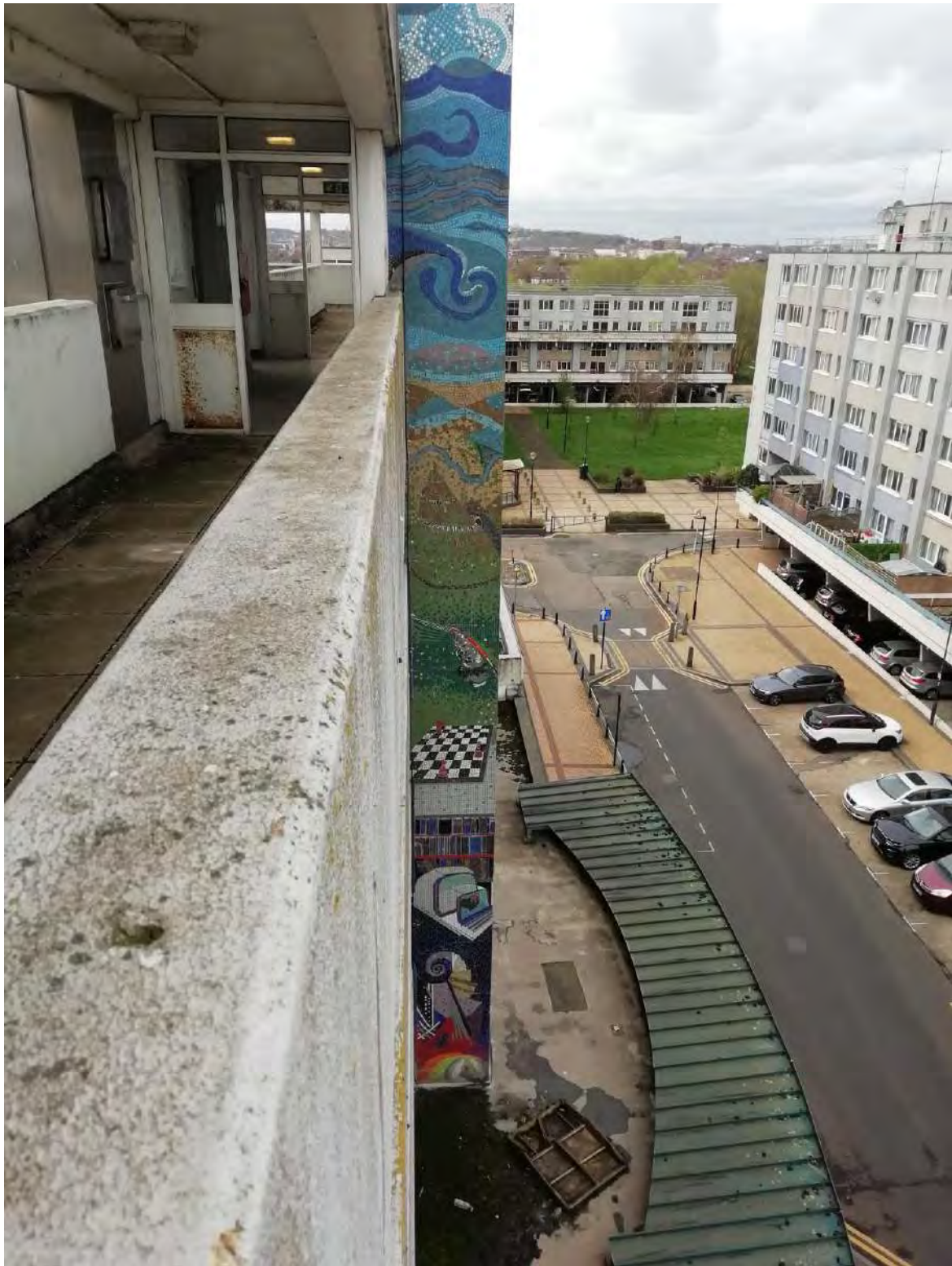
6 th Floor Level – Viewed from Walkway
