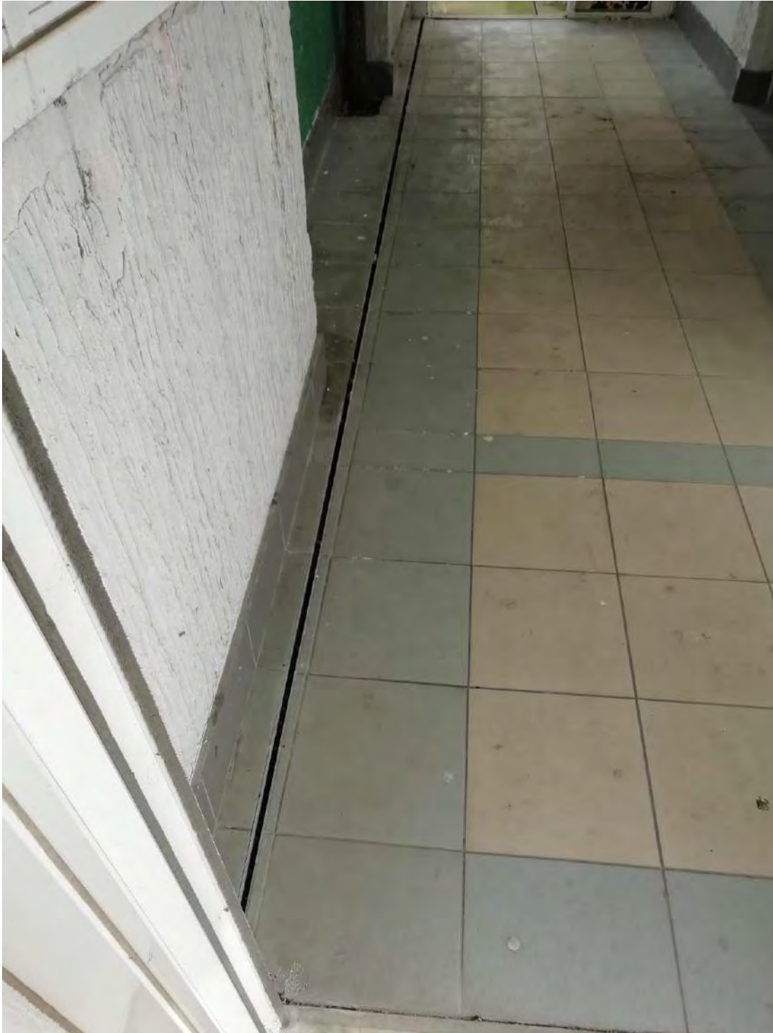
Landing Slab/Walkway Junction
