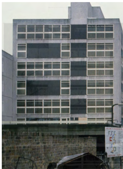
1988 - Before Re-Cladding The steel frames sit up against the blank areas of the facade. The blank areas appear to be painted separating them from the core.
