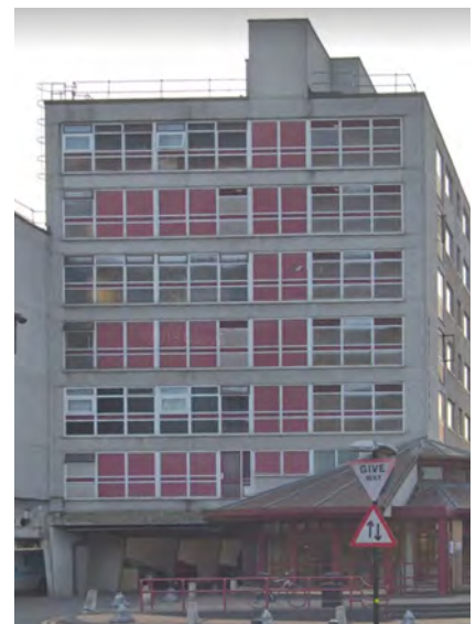
Current The 1990s uPVC windows now sail past the blank areas of the facade covering the areas in coloured spandrel panels.
