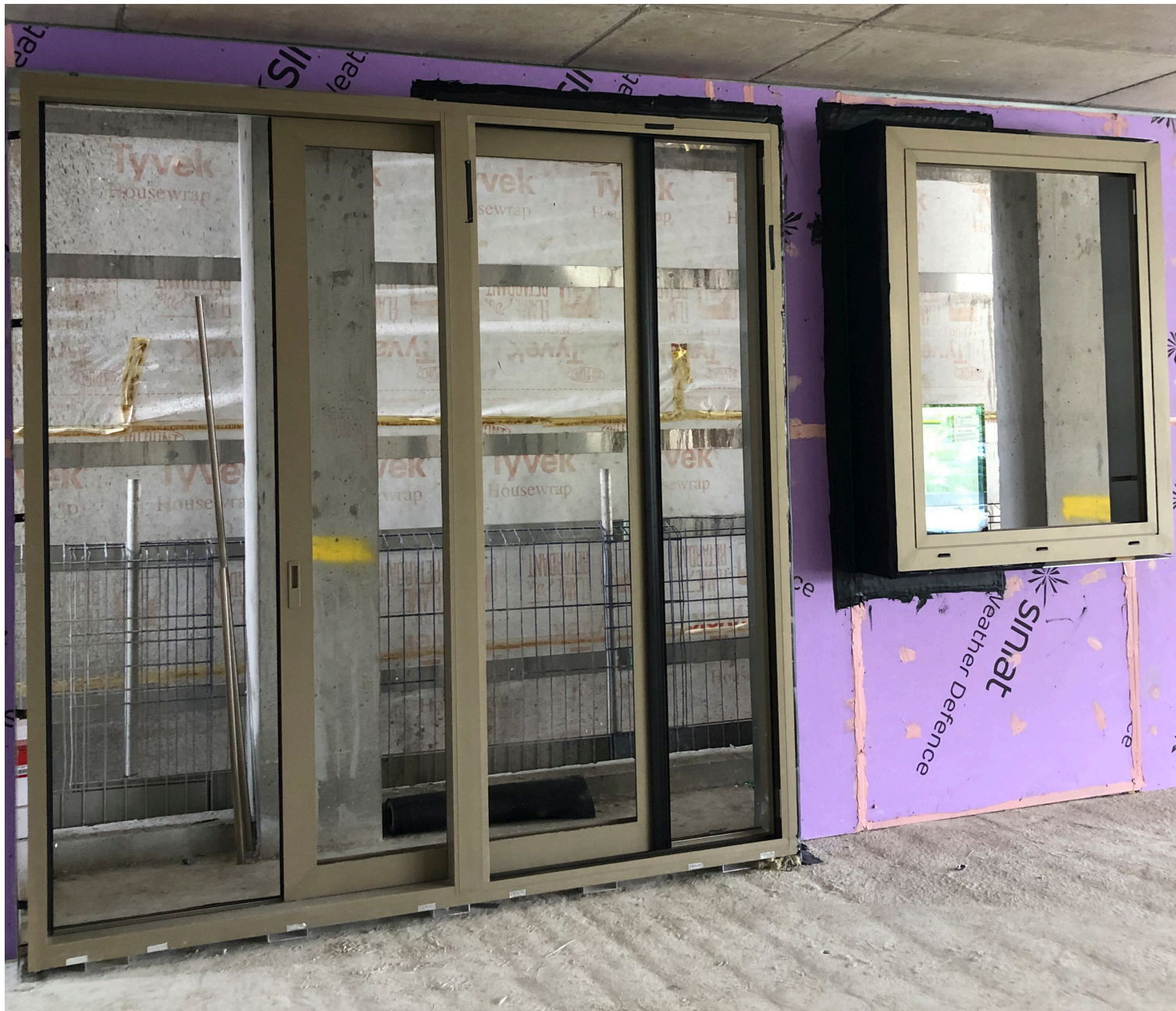
Sliding door and window mock-up
