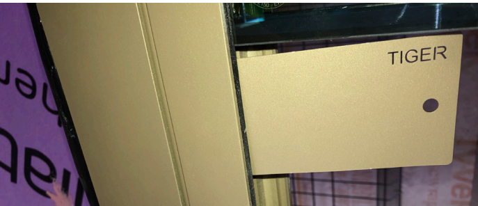
Metal window frame - artificial light (indirect)
