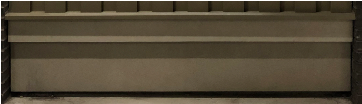
GRC sill and lintel (indirect artificial light)
