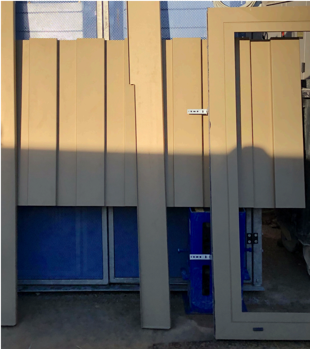
Rainscreen elements and window frame in daylight
