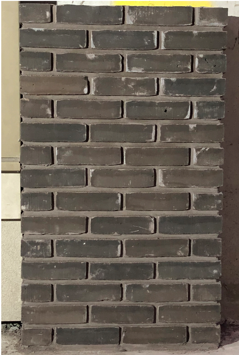
Brickwork sample panel with raked pointing (artificial direct light)
