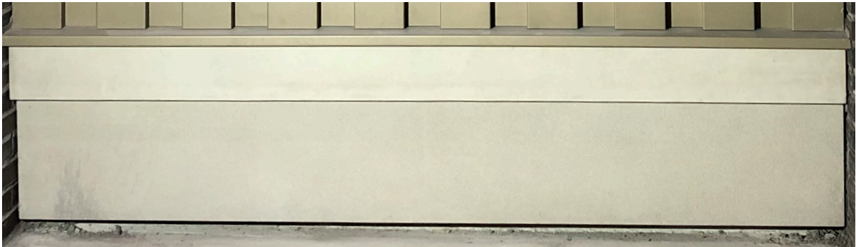
GRC sill and lintel (direct artificial light)
