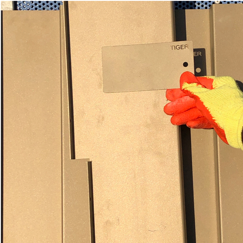
Metal sill and profiled spandrel in daylight
