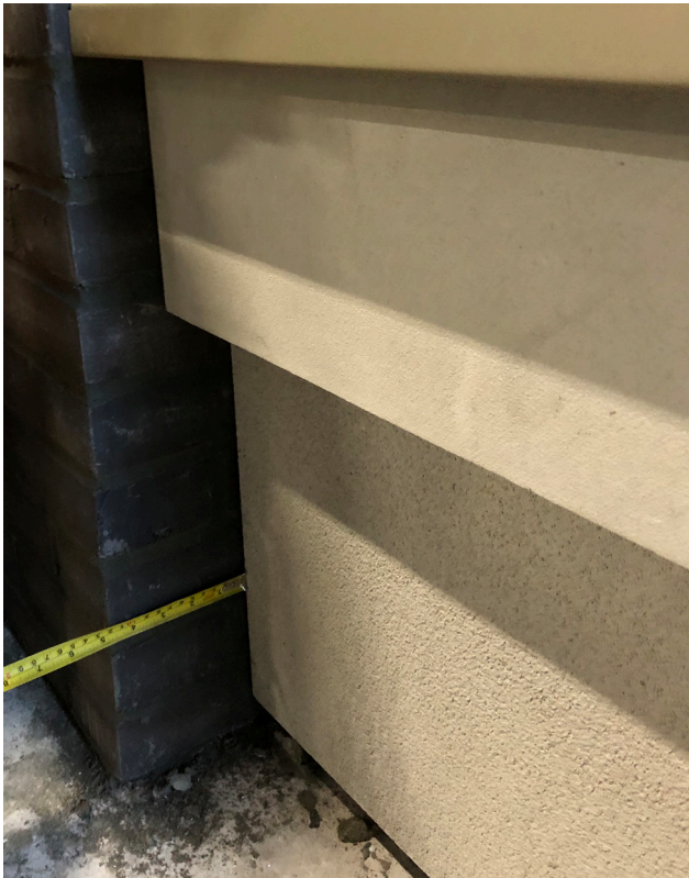
Smooth GRC sill and textured GRC lintel
