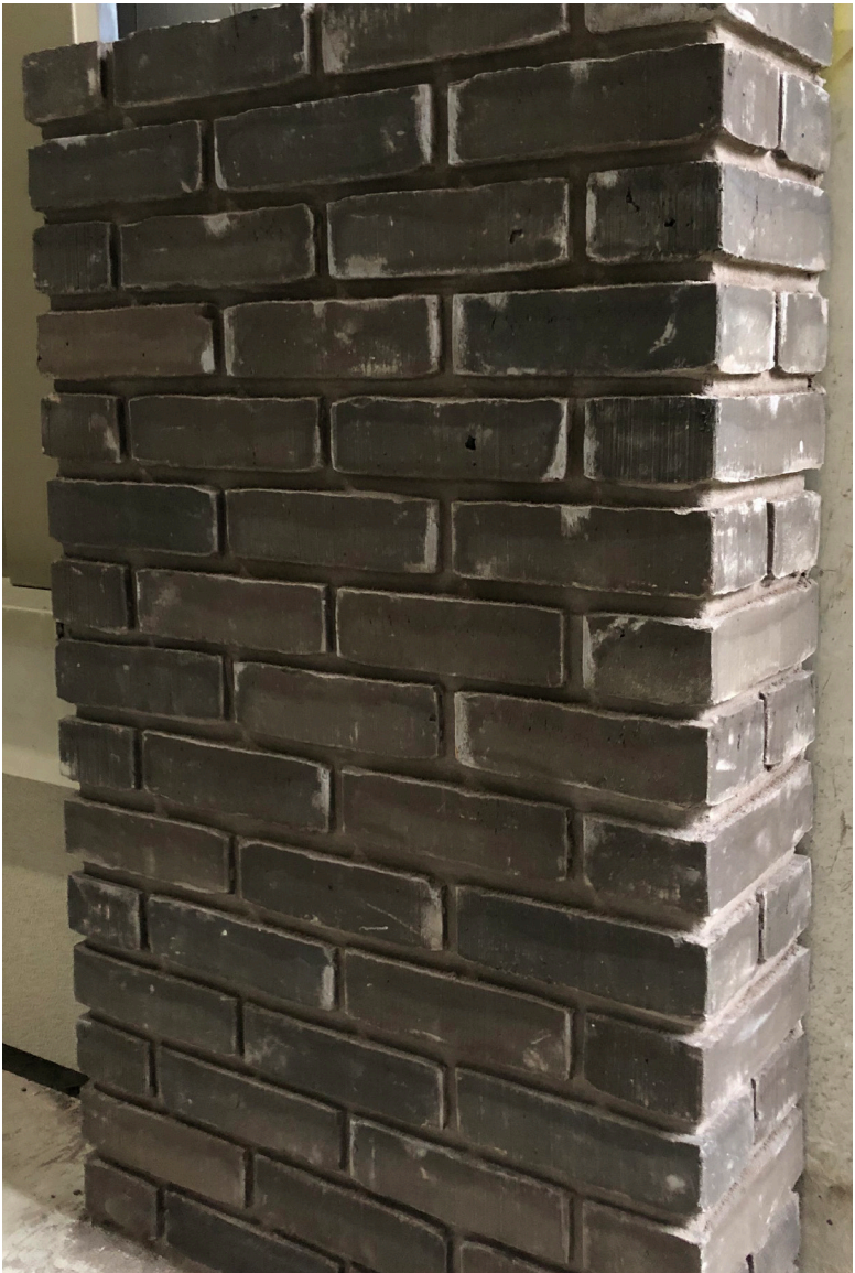
Brickwork sample panel with raked pointing (artificial indirect light on the face and indirect sunlight on the pier return)
