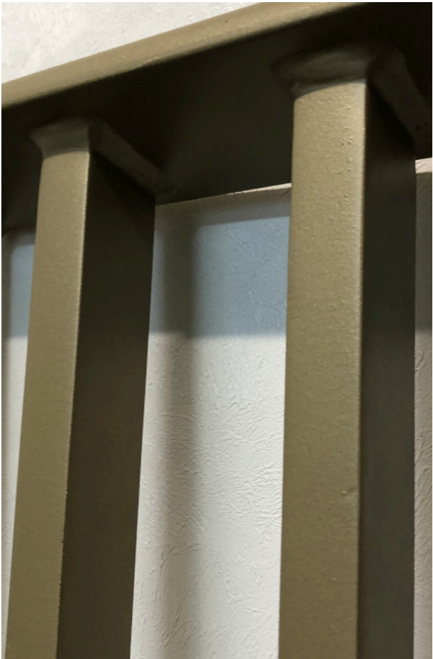
Zoomed-in picture of the proposed balustrade sample. Fin dimension: 20x30mm. Balustrade finish: TIGER Drylac 68/15235
