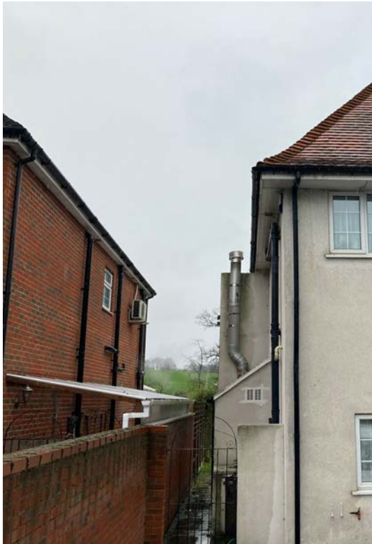
2. Photograph showing the existing gap between 27 and 27A Aylmer Road
