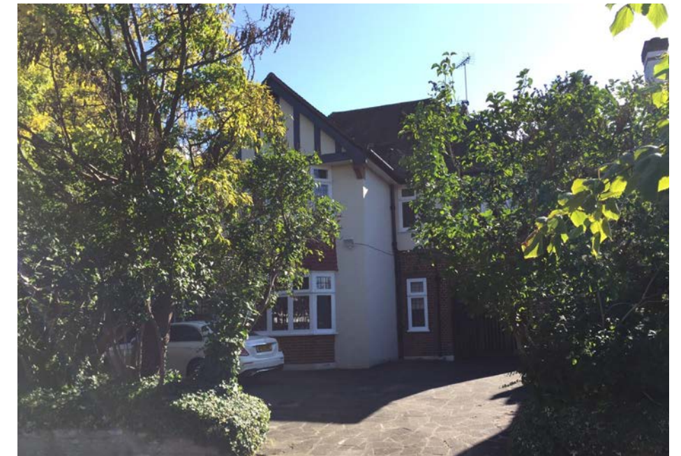
13 Aylmer Road and no.9 appear to have been built to the same original form and design, although each has subsequently been altered in different ways. The main volume of the house has a hipped roof and the two-storey projecting bay on the front elevation has mock-Tudor half-timbering. The form and detailing is inspired by domestic Arts and Crafts architecture and is typical of much inter-war suburban housing. The walls are brick at ground floor and rendered and painted at first floor, with tile hanging details around bay windows.
