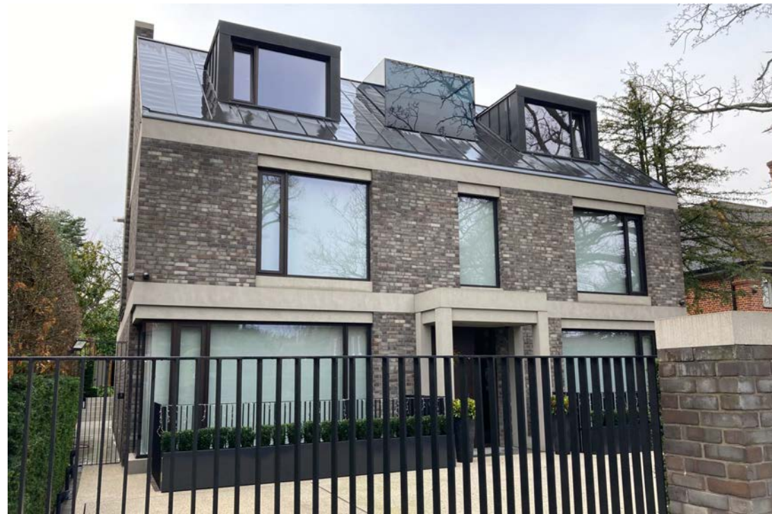
1B Sheldon Avenue. A new house which is unashamedly modern, with a composition that uses classical principles of order. The material palette of grey brick, pre-cast concrete and grey zinc is sharp contrast with its neighbours yet by its scale and form it fits well within the character of the conservation area. Planning permission ref: HGY/2013/0997
