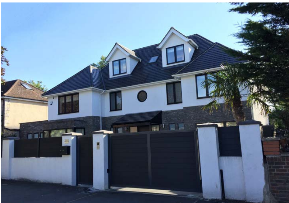
23 Aylmer Road is two doors west of the application site. Haringey Council granted consent for the house to be enlarged and dramatically altered under planning permission ref. HGY/2016/2041. The alterations included over-cladding the original brown brickwork with new grey brickwork at ground floor and white-painted render at first floor, replacing the clay roof tiles with new dark grey roof tiles, installing new dark grey aluminium-framed windows and installing gabled dormers at both front and rear. The result has given the no.23 the appearance of a brand-new house.
