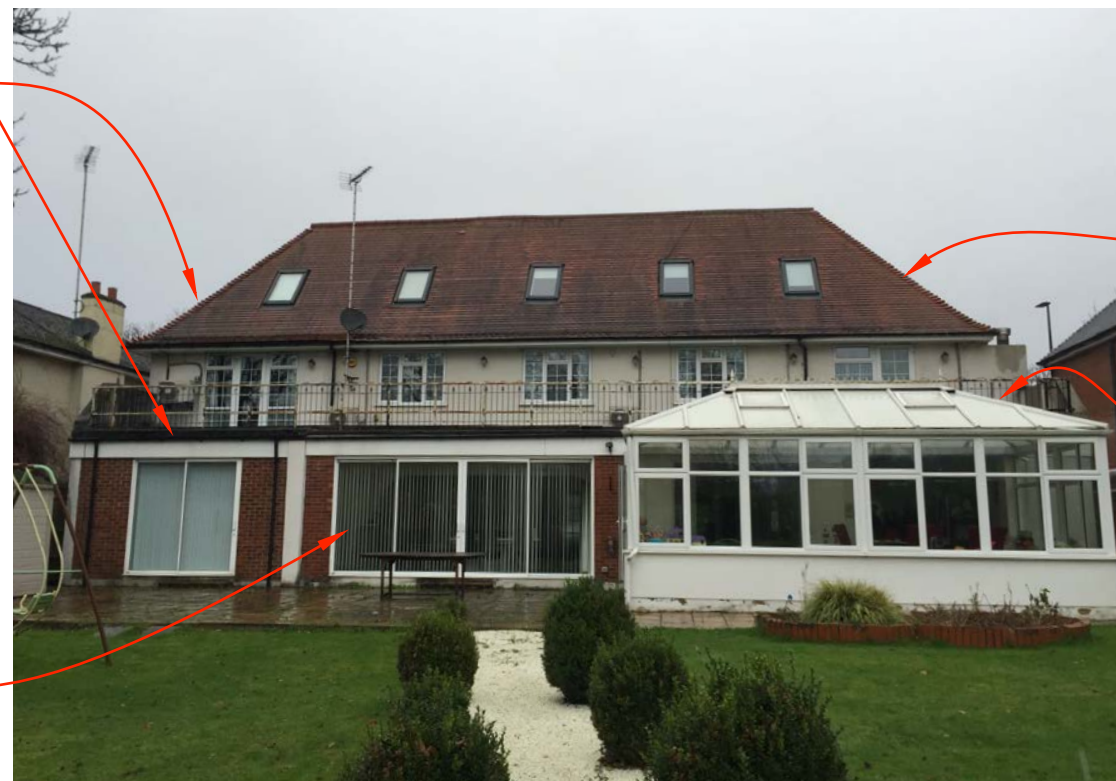
2. Rear Elevation viewed from the rear garden
