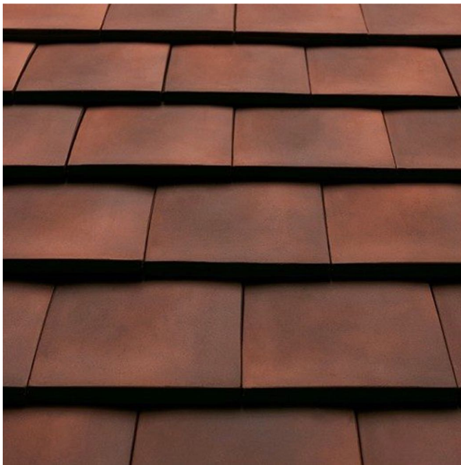
1. Clay roof tiles to the pitched roofs
