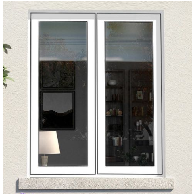
2. Aluminium framed windows, powder coated white with high-performance double glazing
