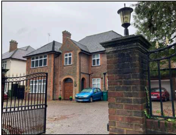
Figure 14. Front elevation of 15 Aylmer Road
