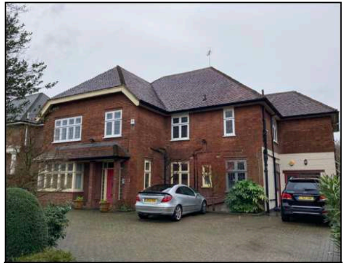
Figure 8. Front elevation of 3 Aylmer Road
