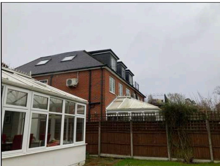
Figure 19. Rear elevation of 27a Aylmer Road as seen from the garden at no. 27
