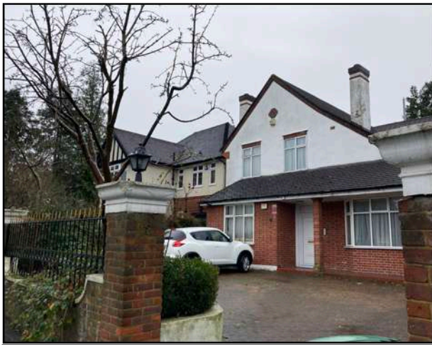
Figure 12. Front elevation of 11 Aylmer Road
