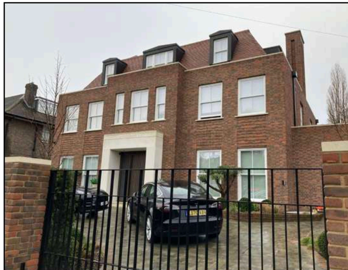
Figure 24. 55 Sheldon Avenue Front Elevation
