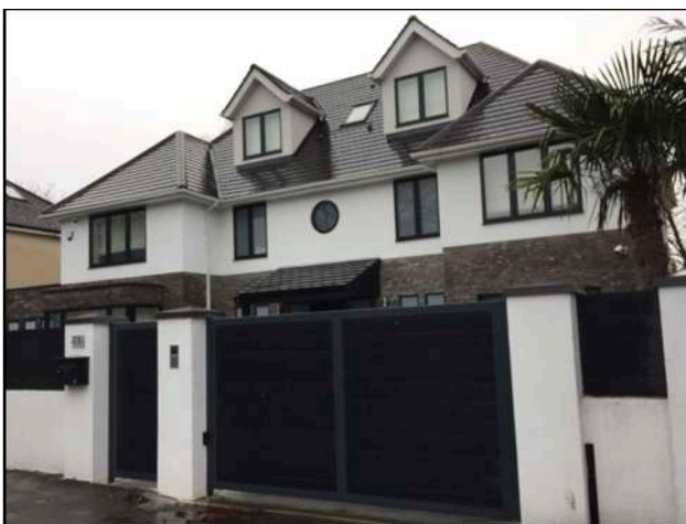
Figure 17. Front elevation of 23 Aylmer Road
