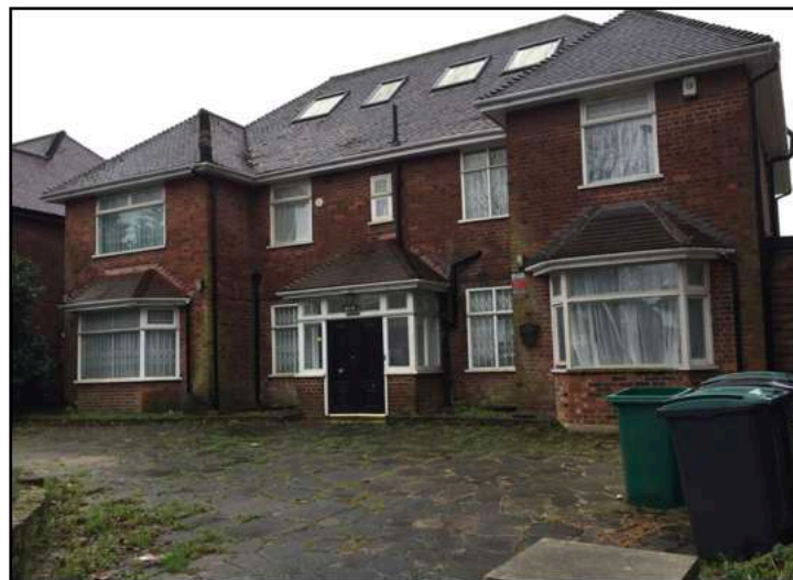
Figure 16. Front elevation of 19 Aylmer Road
