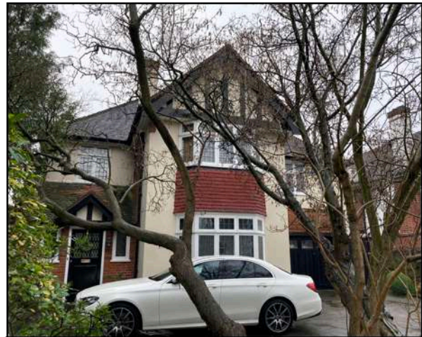
Figure 13. Front elevation of 13 Aylmer Road
