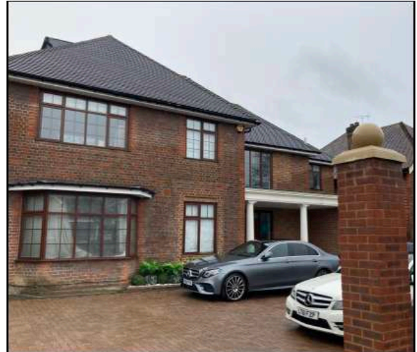
Figure 10. Front elevation of 5 Aylmer Road
