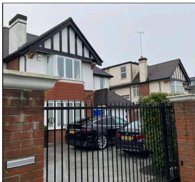
Figure 11. Front elevation of 9 Aylmer Road
