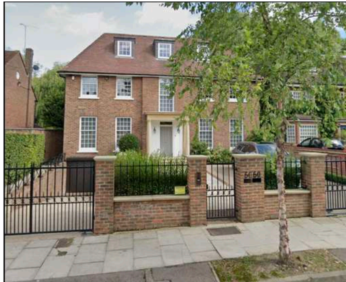
Figure 25. 60 Sheldon Avenue Front Elevation (Source - Google Street View)
