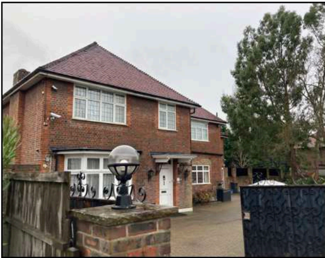
Figure 7. Front elevation of 1 Aylmer Road
