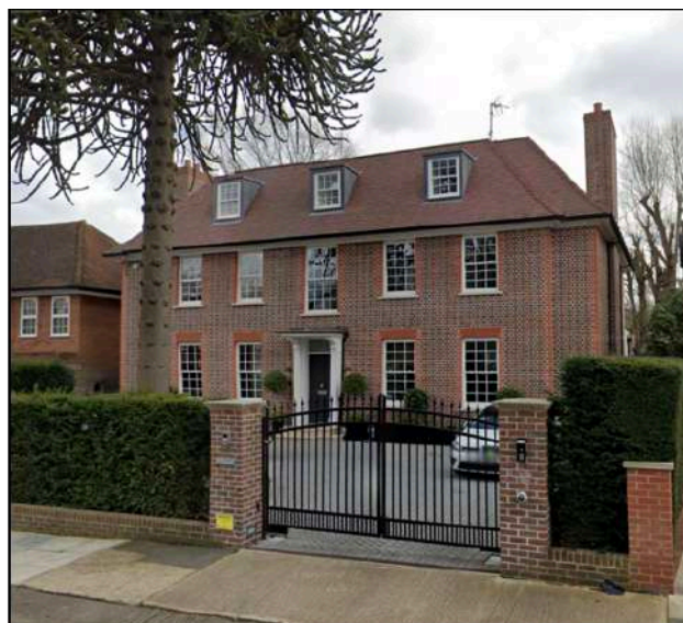
Figure 23. 54 Sheldon Avenue Front Elevation
