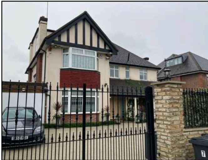
Figure 9. Front elevation of 7 Aylmer Road
