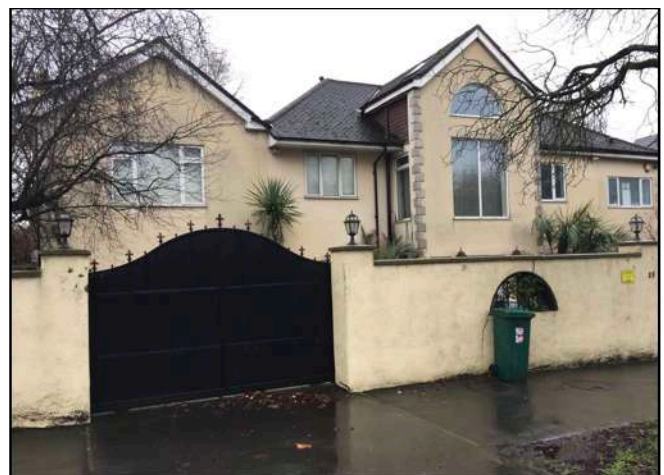
Figure 18. Front elevation of 25 Aylmer Road
