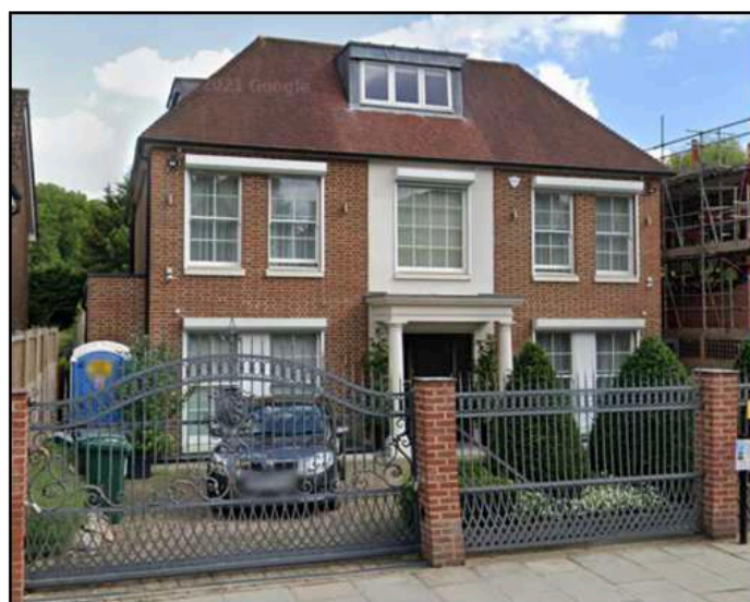
Figure 26. 66 Sheldon Avenue Front Elevation (Source - Google Street View)
