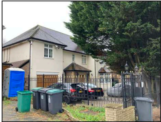
Figure 15. Front elevation of 17 Aylmer Road
