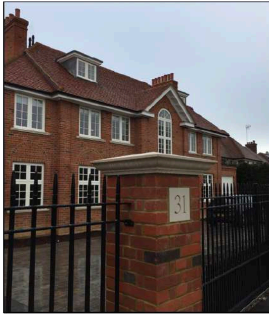
Figure 22. 31 Sheldon Avenue Front Elevation
