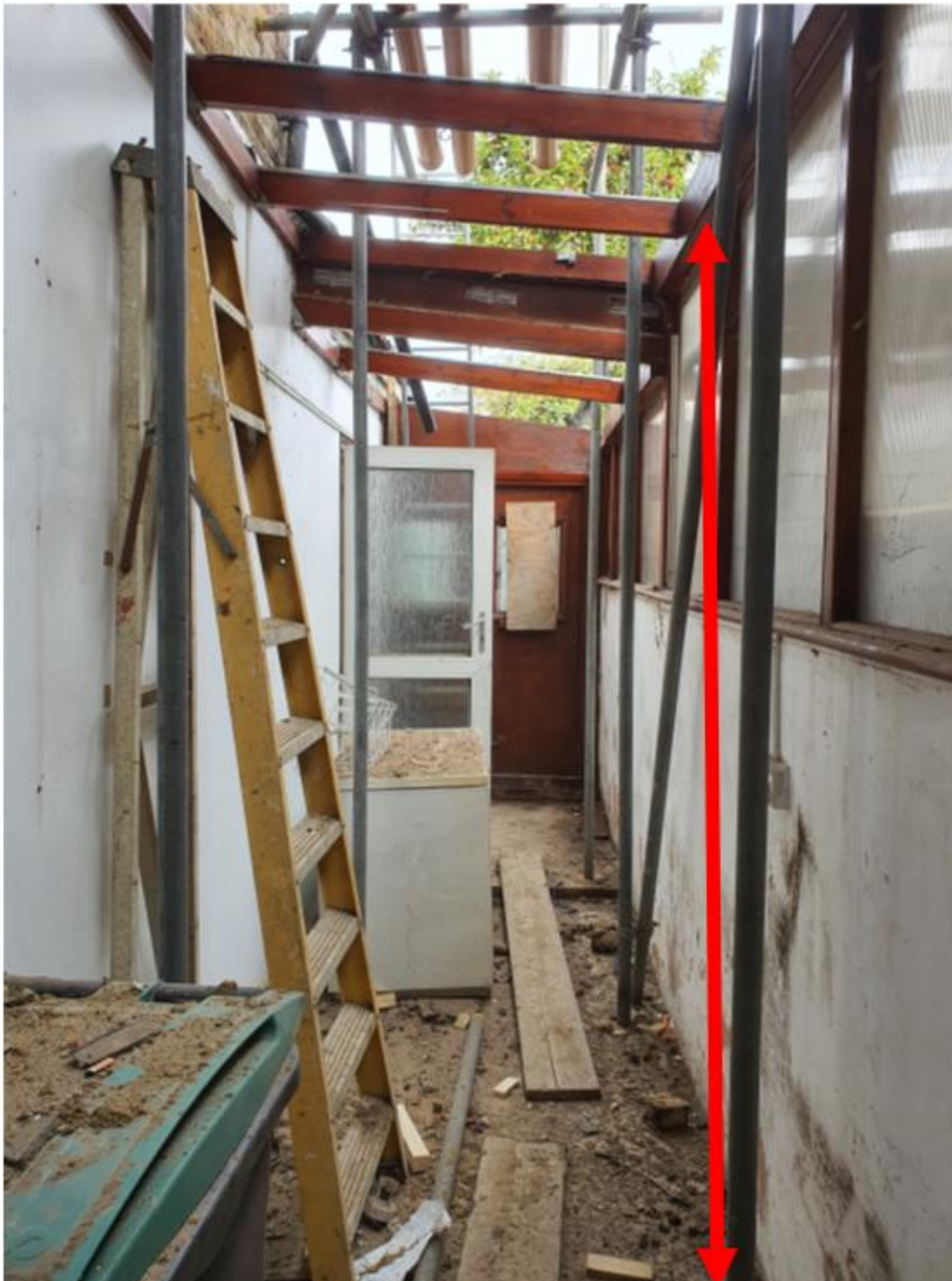
Picture 7. Conservatory – Rear facing to Garden
