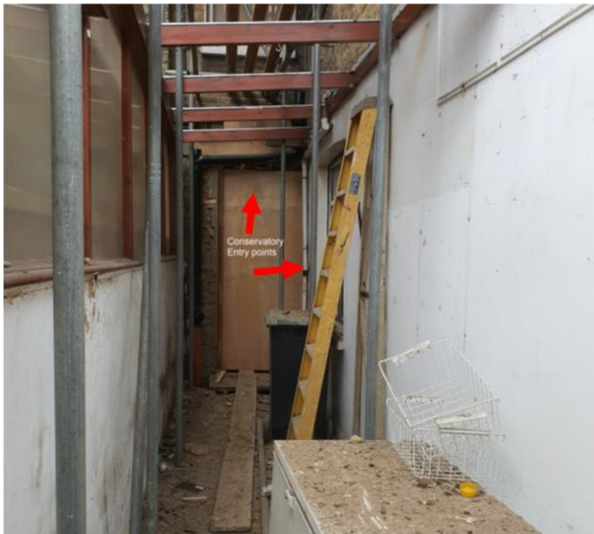
Picture 8. Conservatory – Forward facing toward front of house
