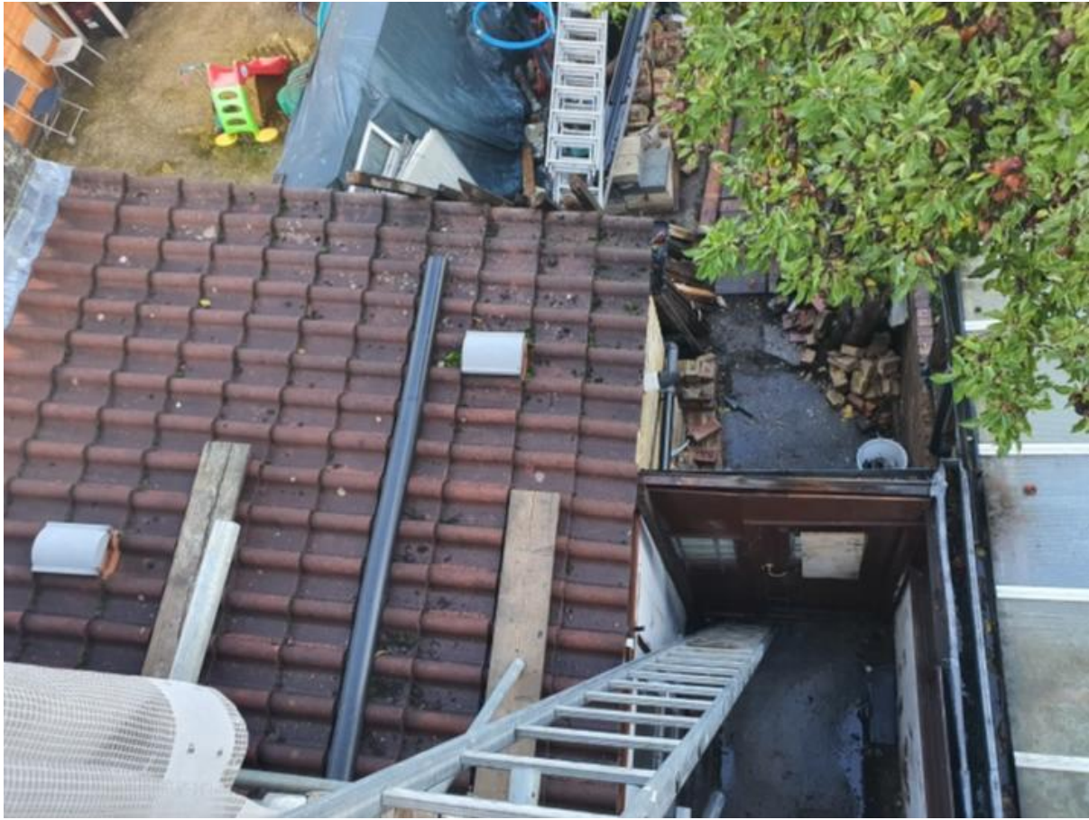
Picture 5. Existing Extension
