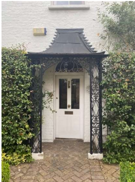
Image 4 – Front porch as existing
