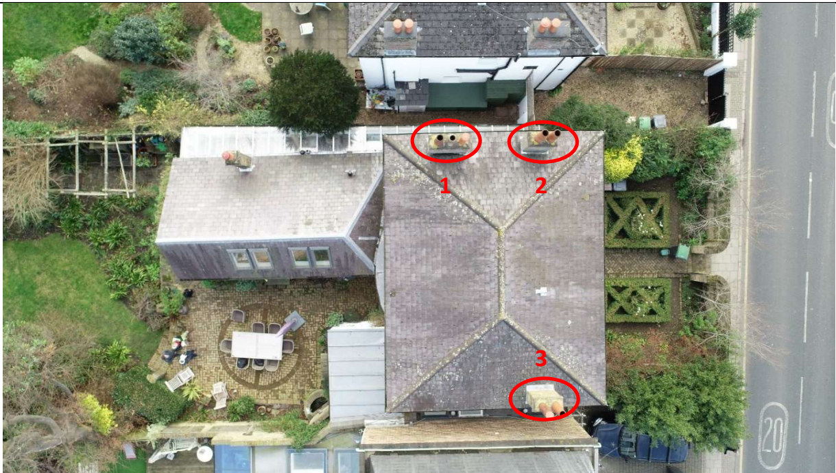
Image 9. Main roof layout with 3nr Chimneys requiring repairs circled in red
