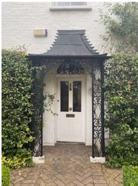
Image 4 – Front porch as existing
