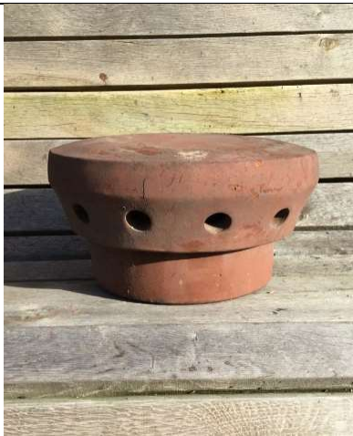
Images 15 & 16- Proposed clay pepperpot ventilation flue for (disused chimney pots) Powder coated metal Terracotta colored rain cowls (active chimneys)
