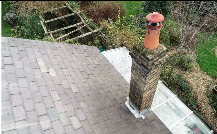
Image 12. Chimney to rear extension with rain cap cowl fitted. (No works required)
