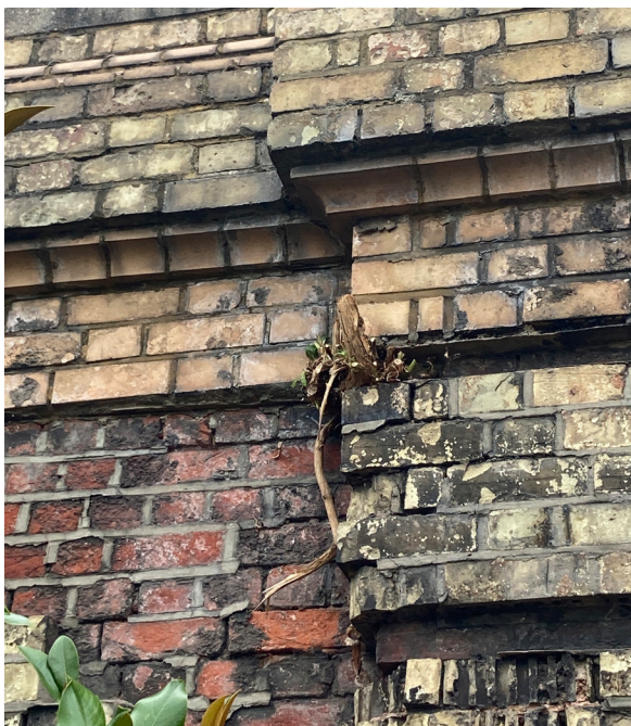
Figures 2 & 3: Examples of brickwork and render repairs required to Traitor's Gate elevation
