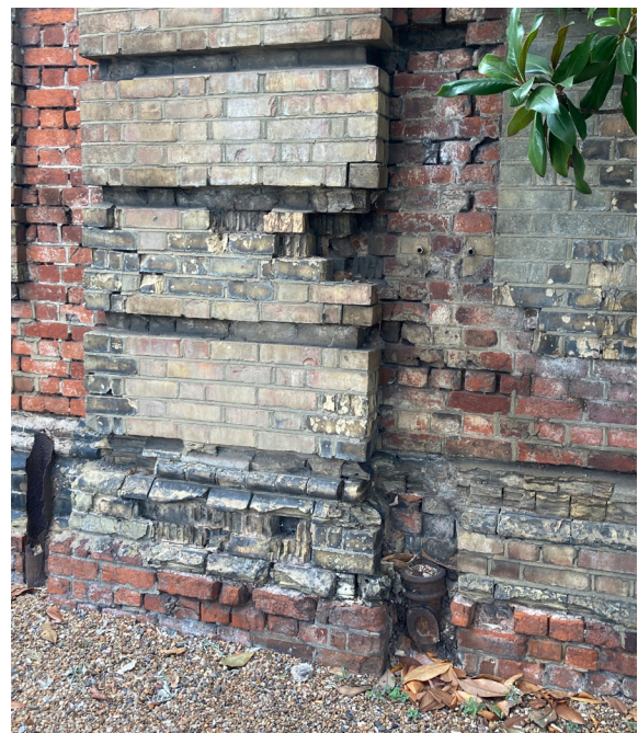
Figures 2 & 3: Examples of brickwork and render repairs required to Traitor's Gate elevation
