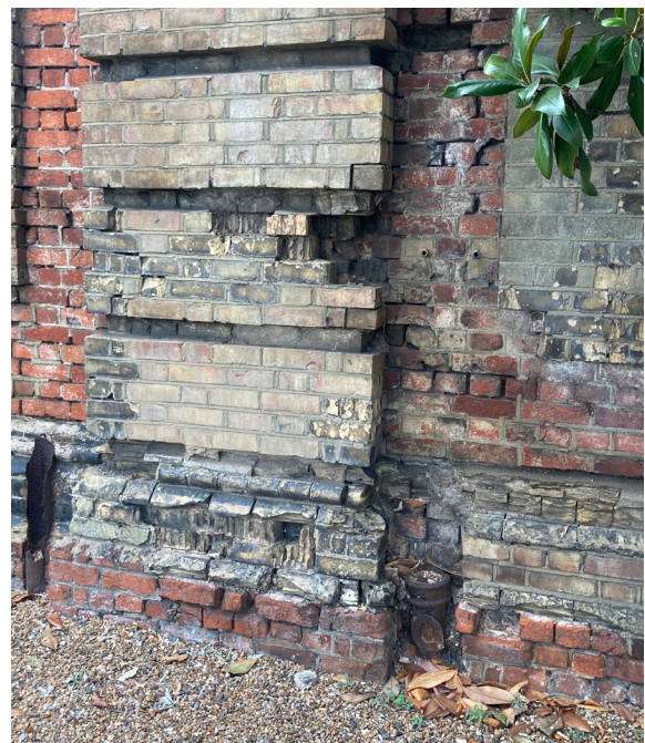
Figure 4,5 & 6: Examples of brickwork and render repairs required to Traitor's Gate elevation
