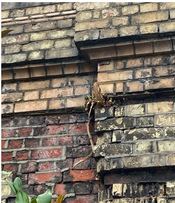
Figure 4,5 & 6: Examples of brickwork and render repairs required to Traitor's Gate elevation
