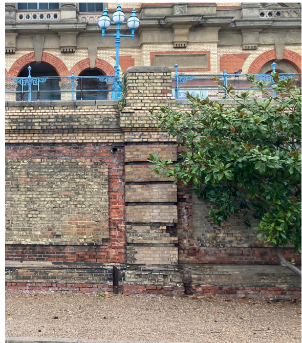
Figure 1,2 & 3: Examples of brickwork and render repairs required to Traitor's Gate elevation
