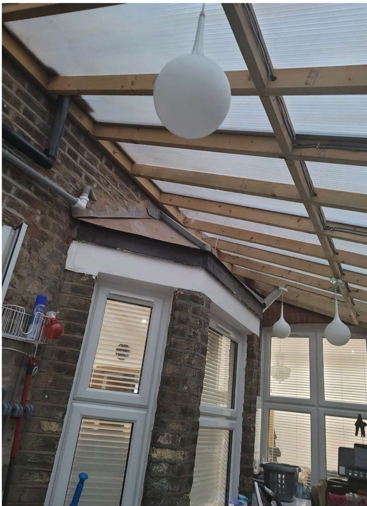
Inside Temporary lean-to
