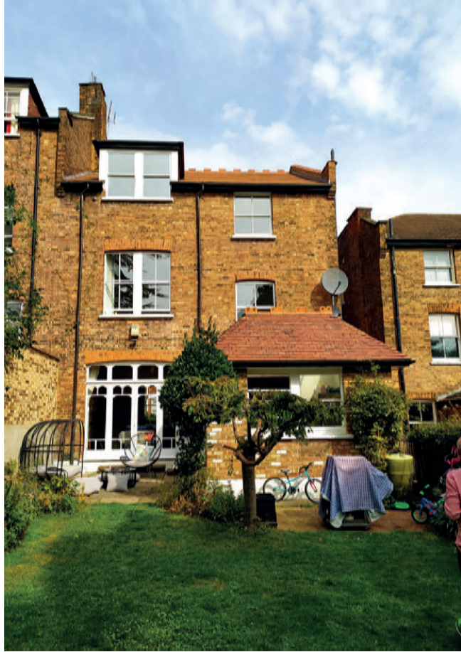
View of the existing rear elevation from the rear garden showing the scale of the existing rear extension.
