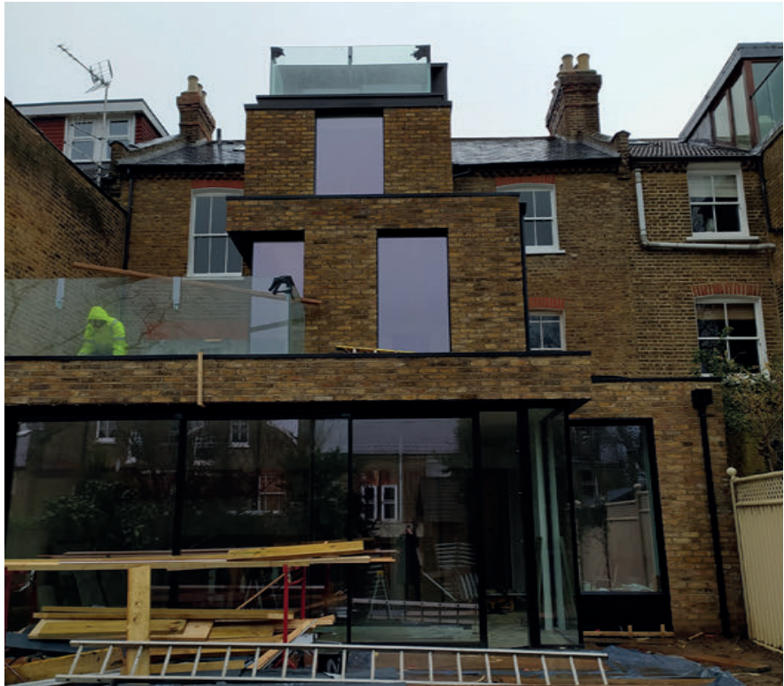
Mount View Road N4 completed under former name of Clarke Penman Ref: HGY/2019/2279 10/10/2019
