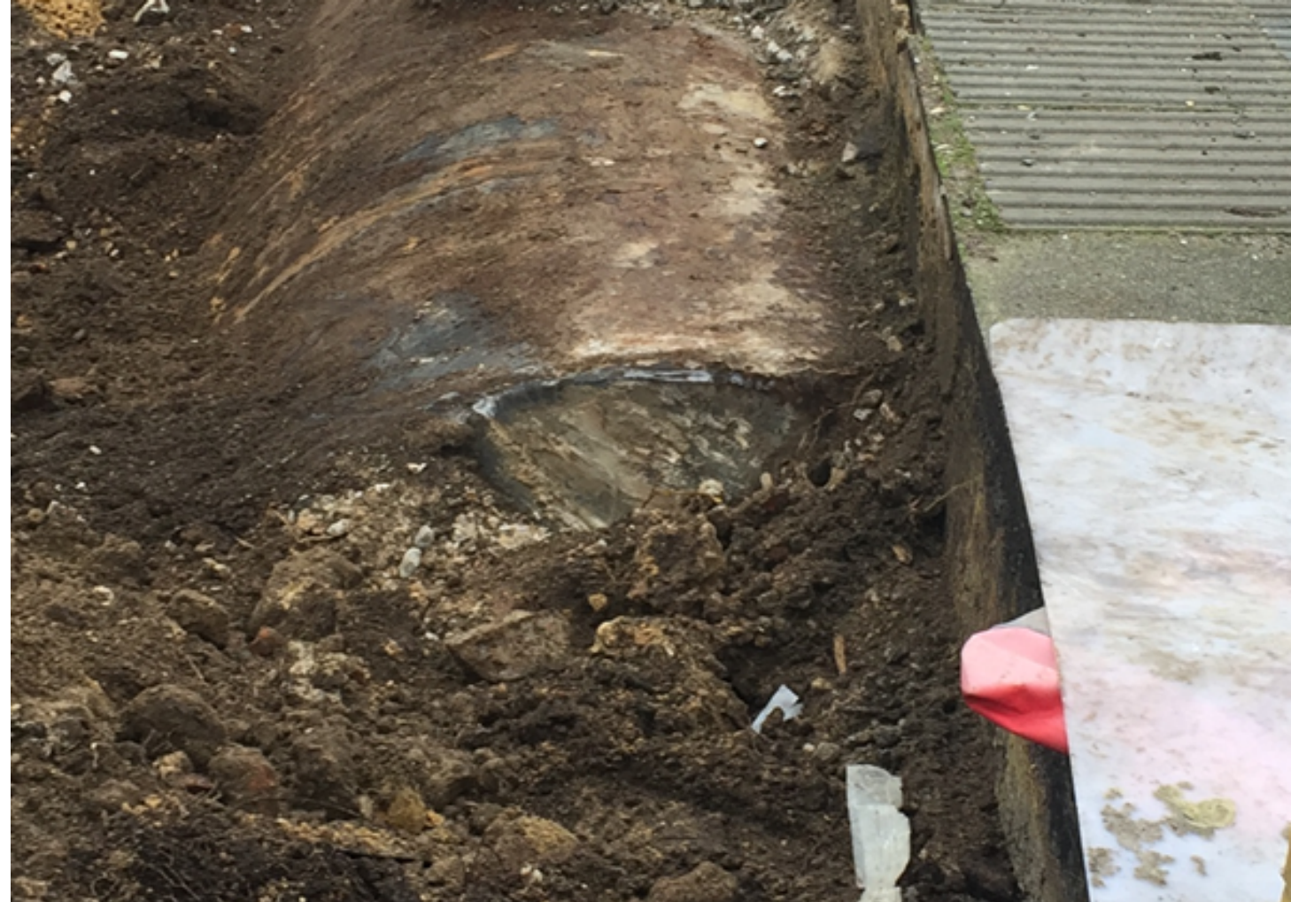
Photos of underground storage tanks uncovered during site investigation undertaken in 2020. Photos taken from Langan Geo-Environmental Site Assessment Report 4th November 2021
