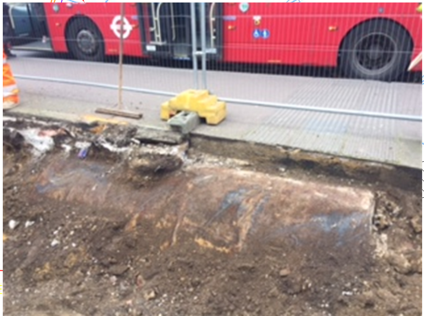
Photos of underground storage tanks uncovered during site investigation undertaken in 2020. Photos taken from Langan Geo-Environmental Site Assessment Report 4th November 2021
