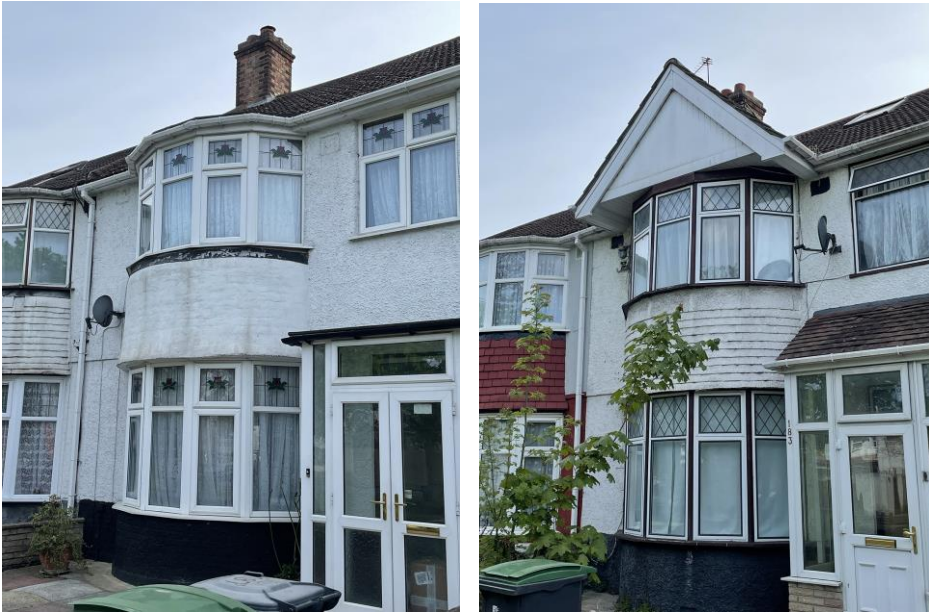
Img 3 & 4. Other front Elevations on Downhills Way.
