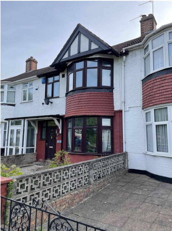
Img 1. Main Elevation on Downhills Way
