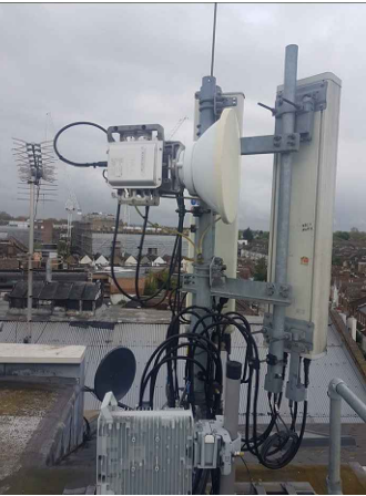
SECTOR 1 FEEDERS TO ANTENNAS NTS
