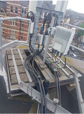
SECTOR 2 FEEDERS TO ANTENNAS NTS
