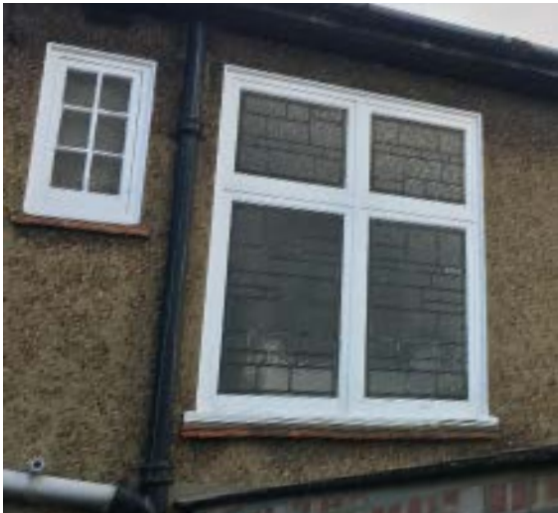
Side Window to staircase to be re-claimed and re used
