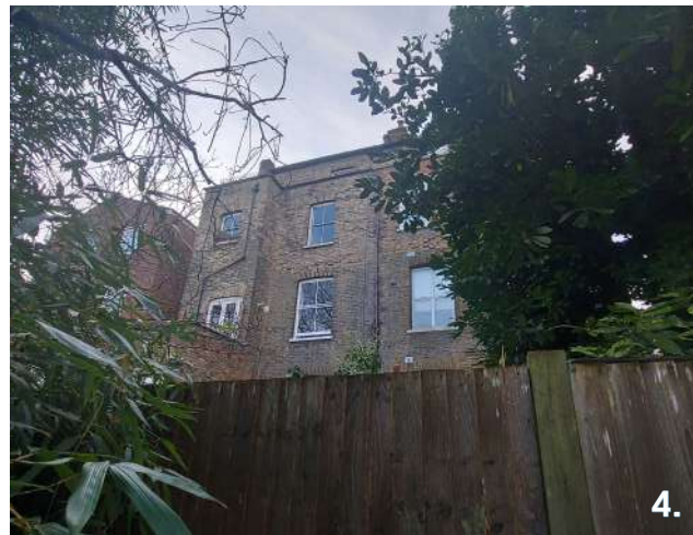
Rear Elevation of the site
