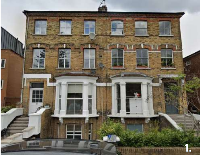
Front Elevation of the site
