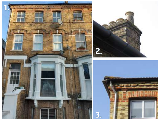
Fig 1-3: Brick detailing to the front elevation and chimney stacks
