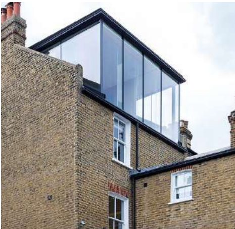
Bolingbroke Grove, MCG Architects
