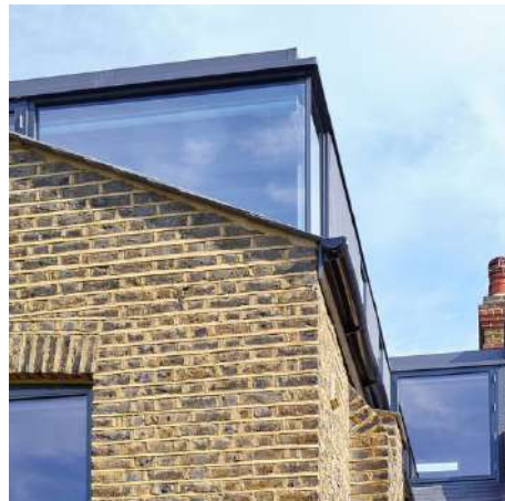
Kennington House, R2 Studio Architects
