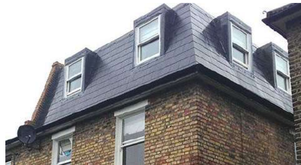
Roof Slate tiles
