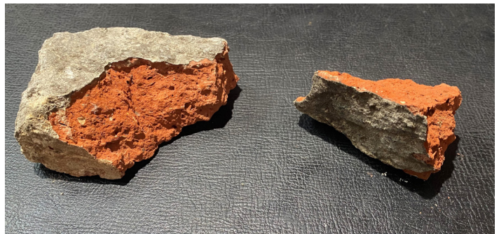
Figure 12- Samples of existing facing bricks from Pier There is a very significant deposit of grey weathering on all exposed surfaces
