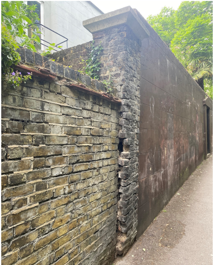
Figure 6 - View from Southwood Lane Looking South (Existing condition)
