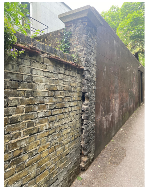
Figure 4 - View from Southwood Lane Looking South (Existing condition)
