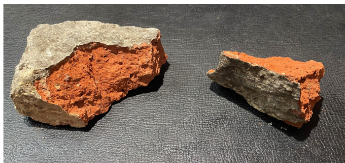
Figure 4 – Samples of existing facing bricks from Pier
