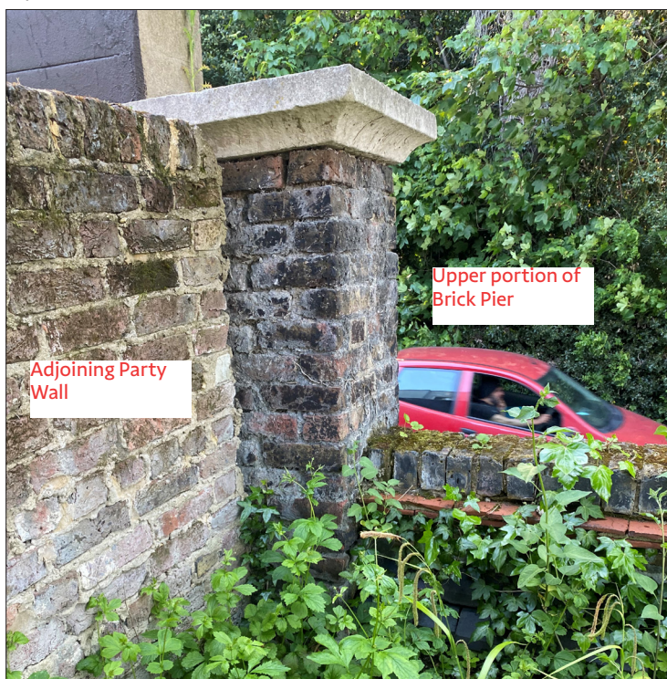
Figure 14 – Photograph showing upper portion of Pier July 2022
