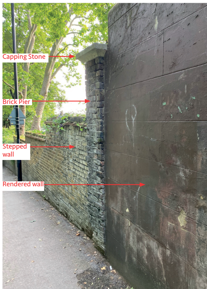
Figure 8 – Photograph of Brick Pier and stepped wall (2022) Taken July 2022 (Photograph by SHERCO)
