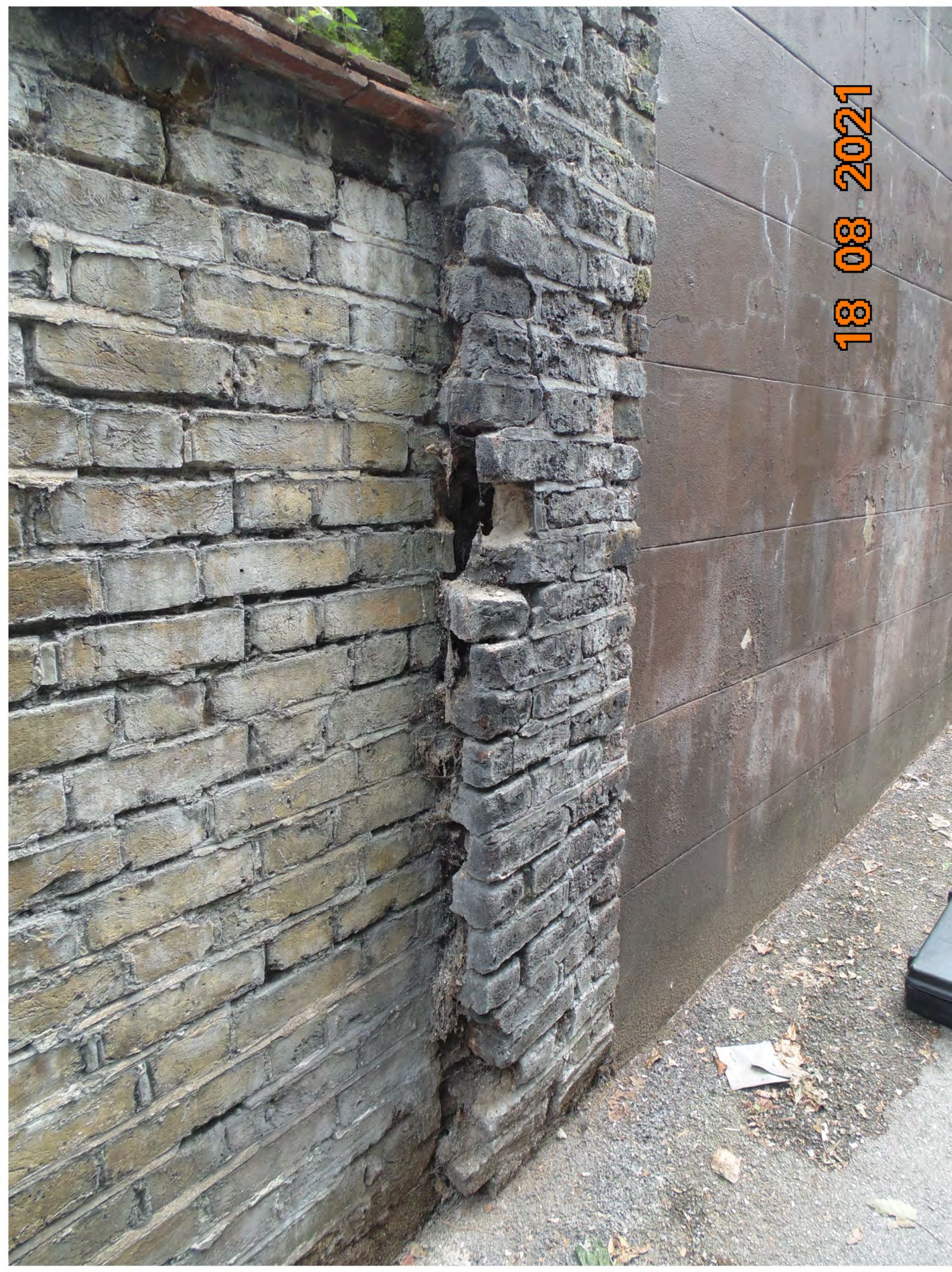
Condition photos of Pier at Southwood Lane Taken 8th July 2022
