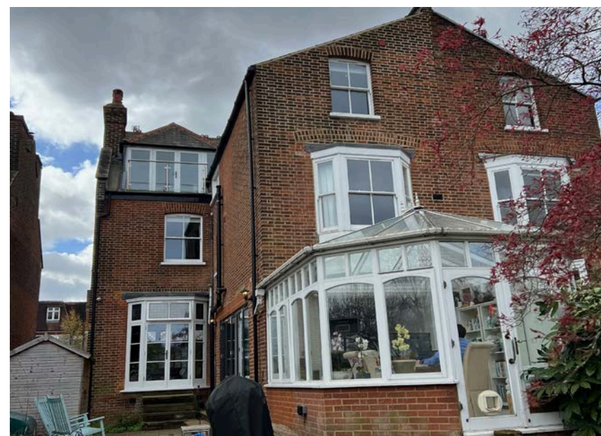
Figure 4.3 Rear of the house
