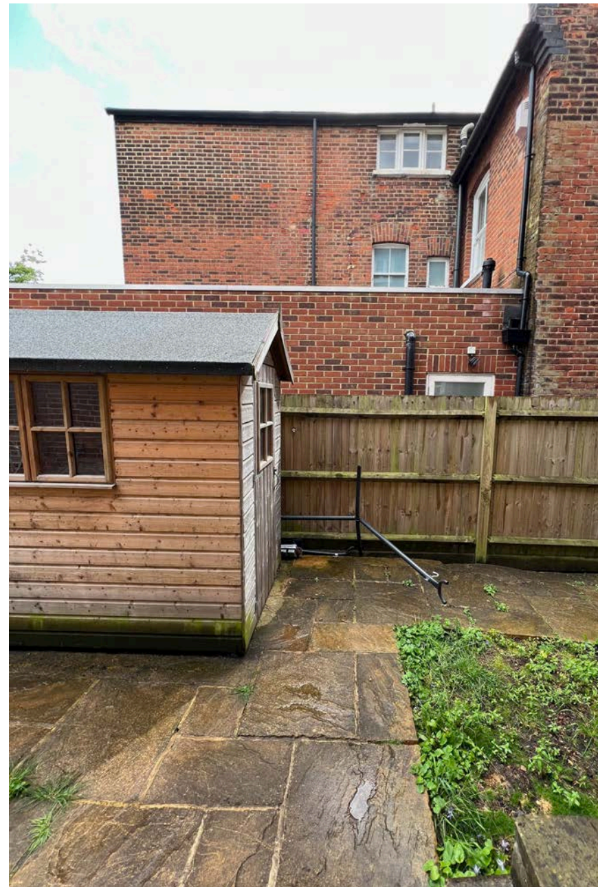
Figure 3.11 Courtyard with neighbour's extension in the background
