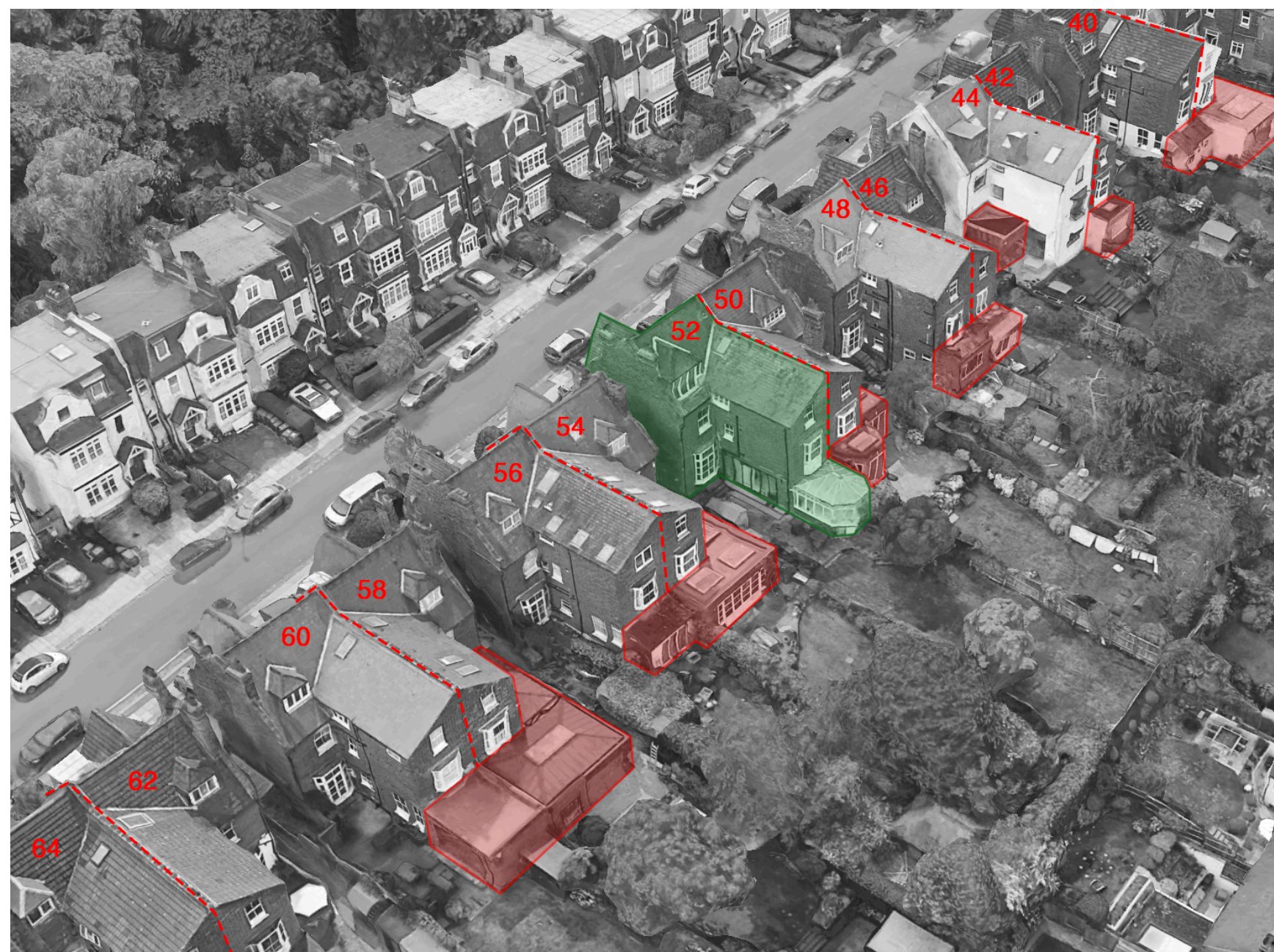
Figure 2.1 52 Onslow Gardens and its neighbouring rear extensions
