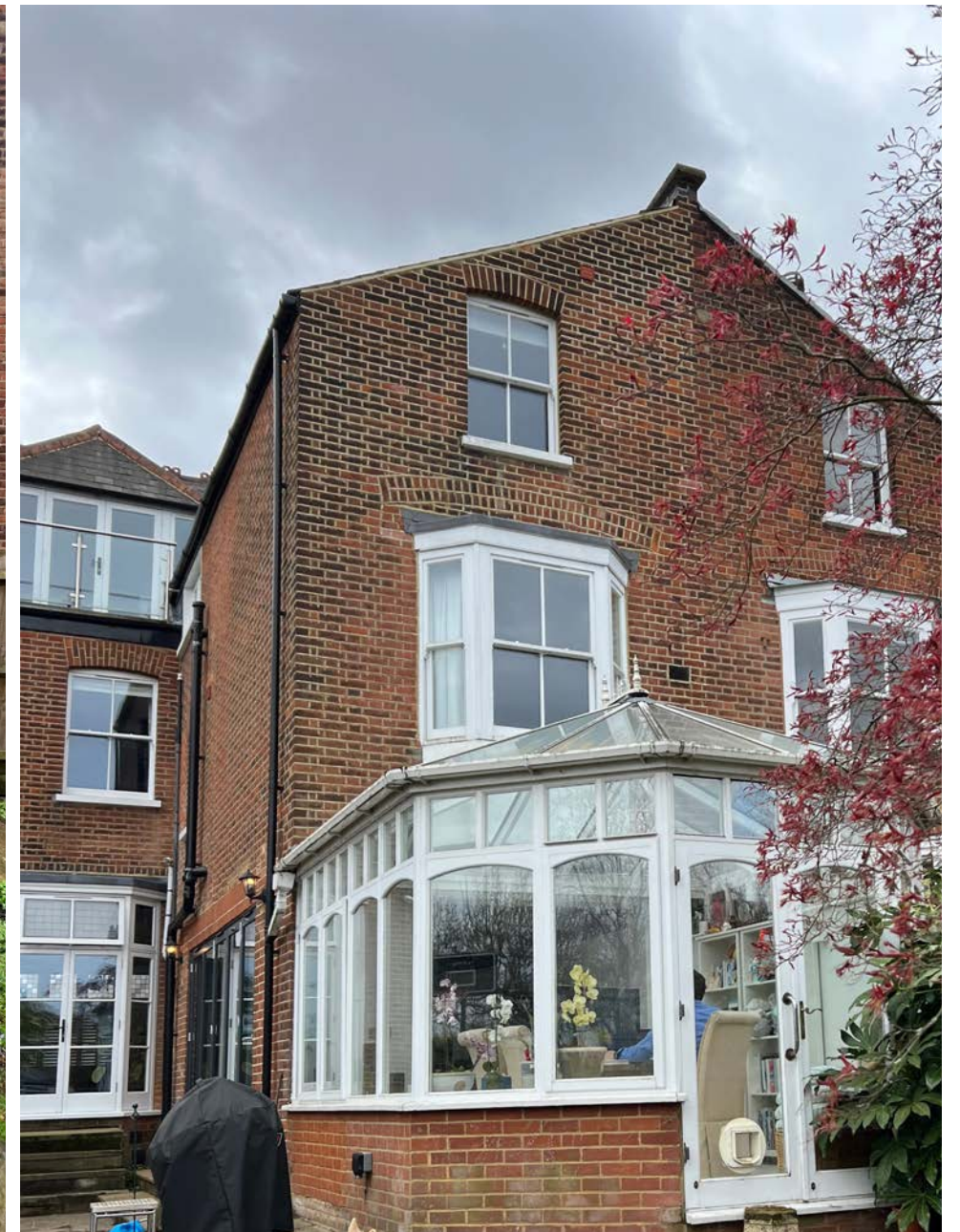
Figure 3.12 Existing rear conservatory
