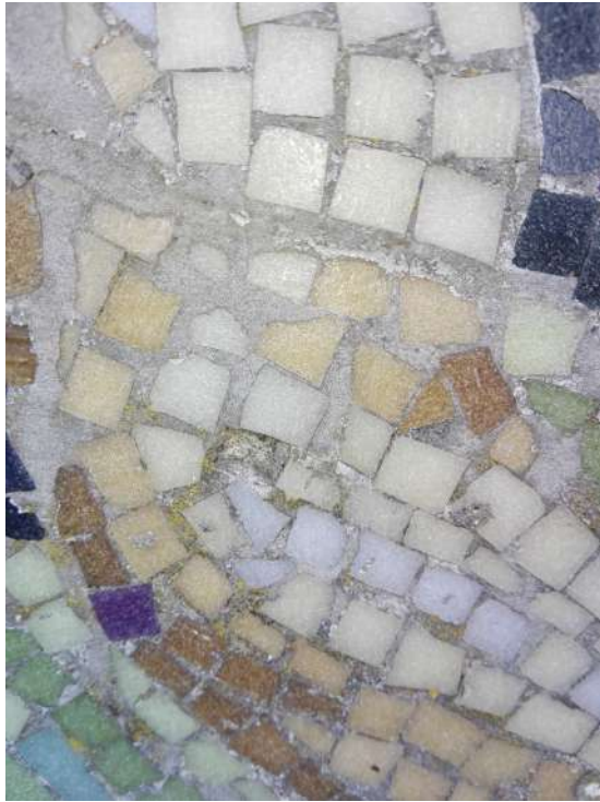
Images 3a-b – “Opaque” effect due to high presence of limescale plus whitening of cement carbonation
