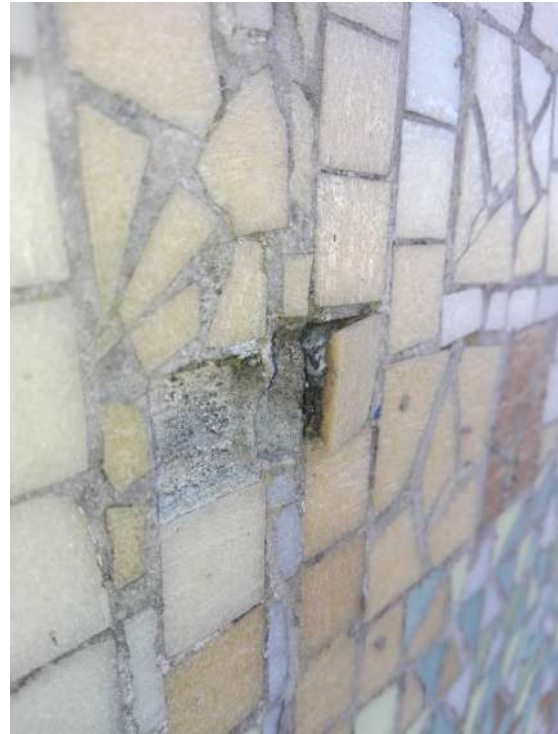
Images 4a-b – Detachment of tesserae from the substrate
