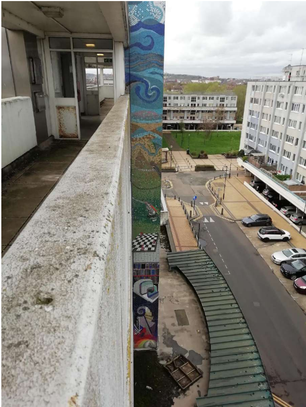
6 th Floor Level – Viewed from Walkway
