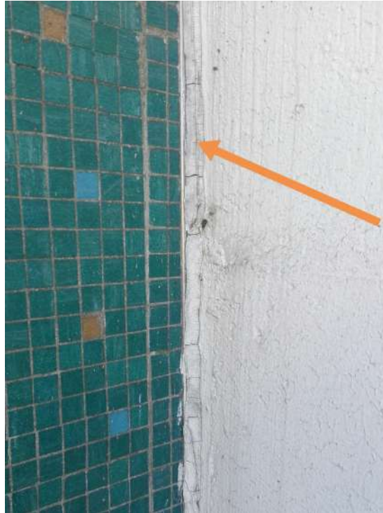
Image 10 – Stainless steel strip along vertical side ends
