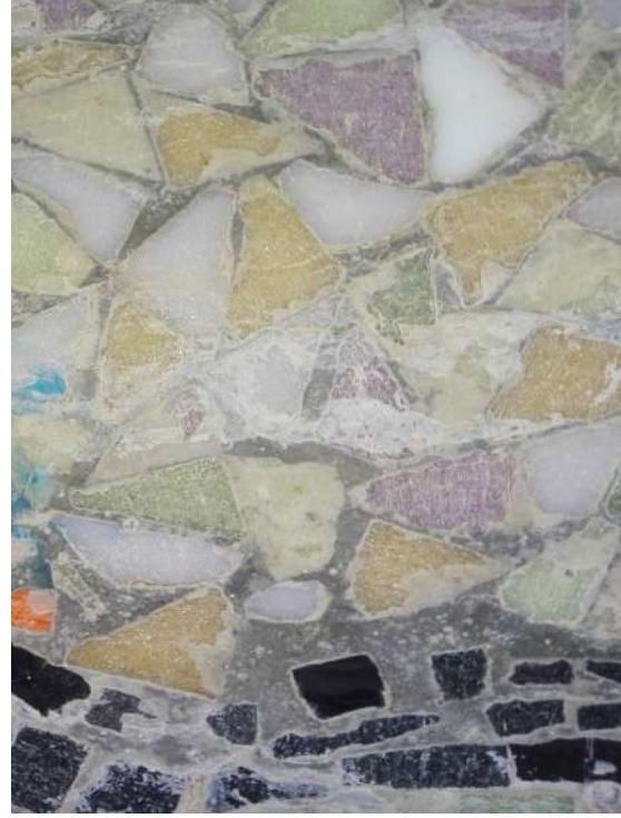
Images 3a-b – “Opaque” effect due to high presence of limescale plus whitening of cement carbonation
