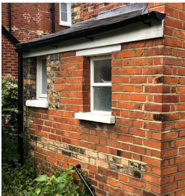
Windows W3 and W4
