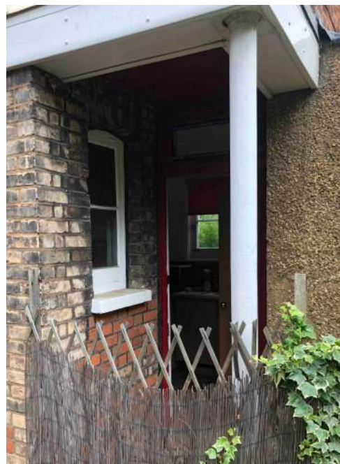
Window W5 and Door D1
