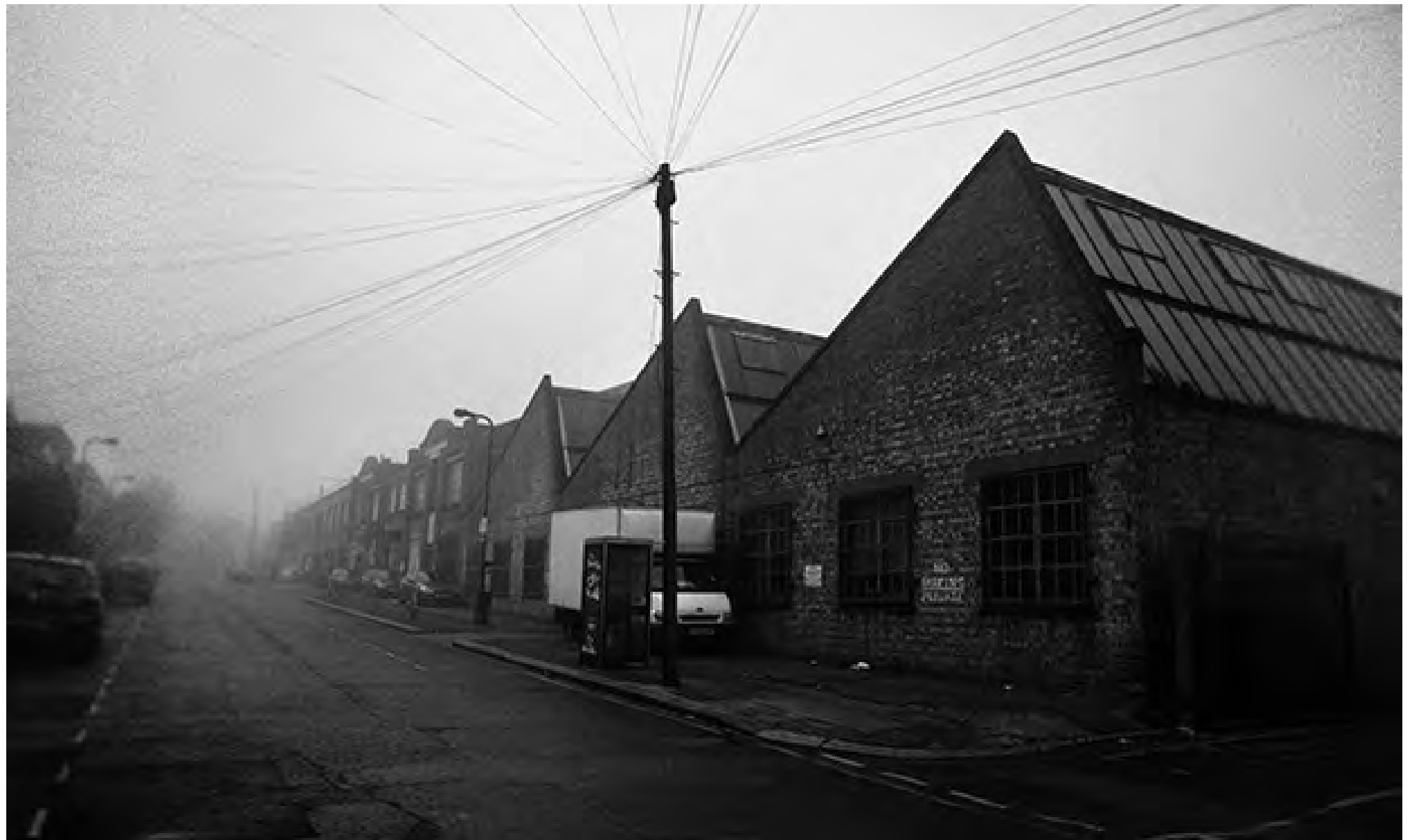
Omega Works from Hermitage Road
