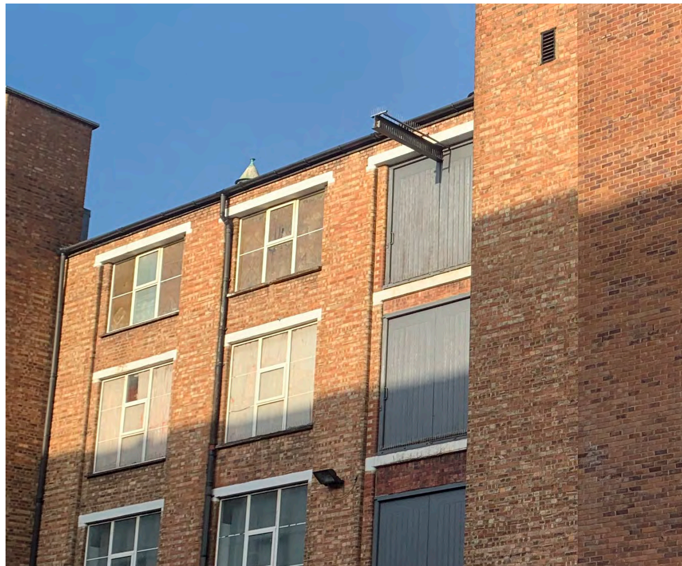
The Oriental Carpet Centre Building, Vale Road
