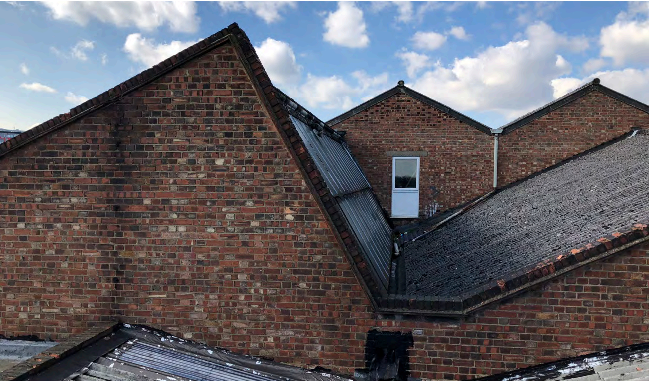
Saw Tooth roof forms of the existing building
