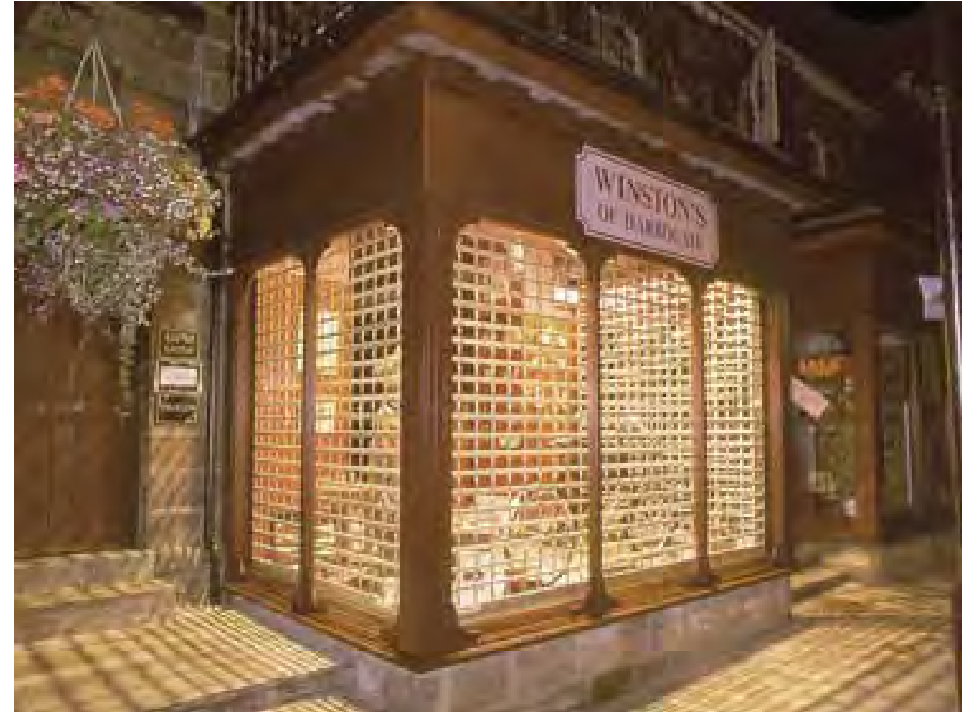
An example of internal security shutters that preserve the detailing of the external facade
