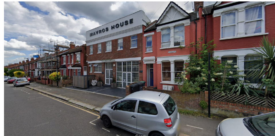
Two storey terraced housing opposite the site
