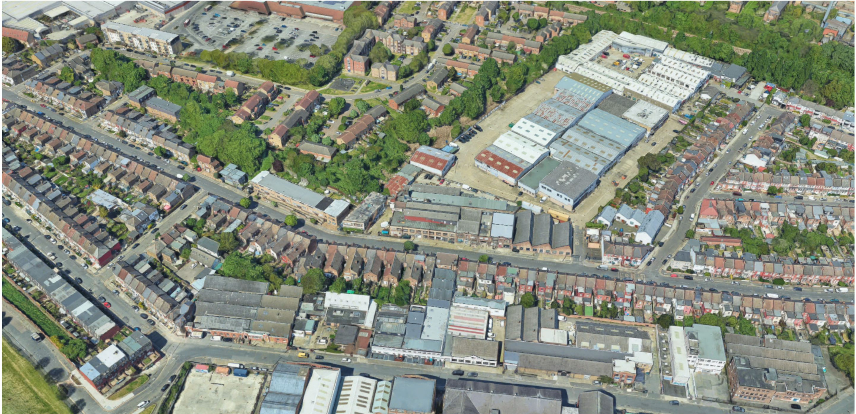
Aerial view of site looking north
