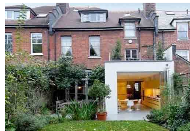
Render extension at 4 Clifton Road with bifold doors
