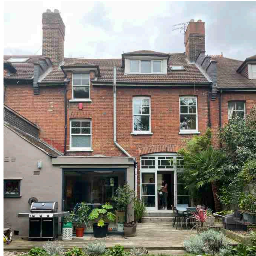
6 Clifton Road - View from behind showing modern extension
