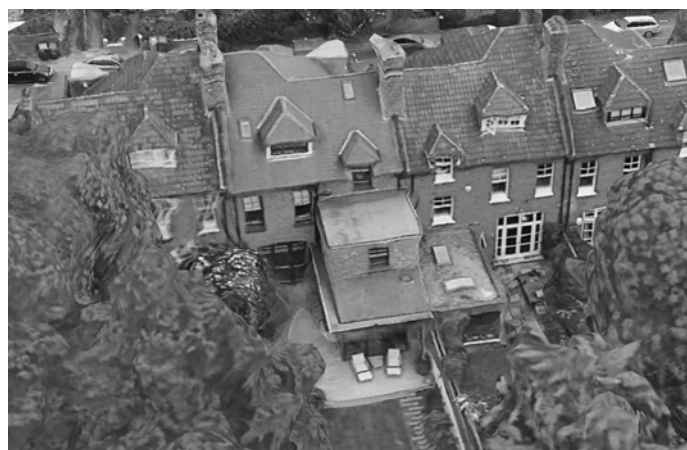
Modern extensions at 10 and 12 Clifton Road
