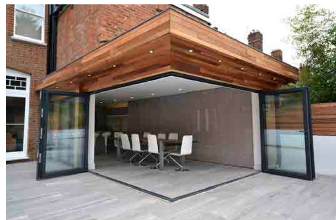
Timber clad extension to 12 Clifton Road with large glazed doors
