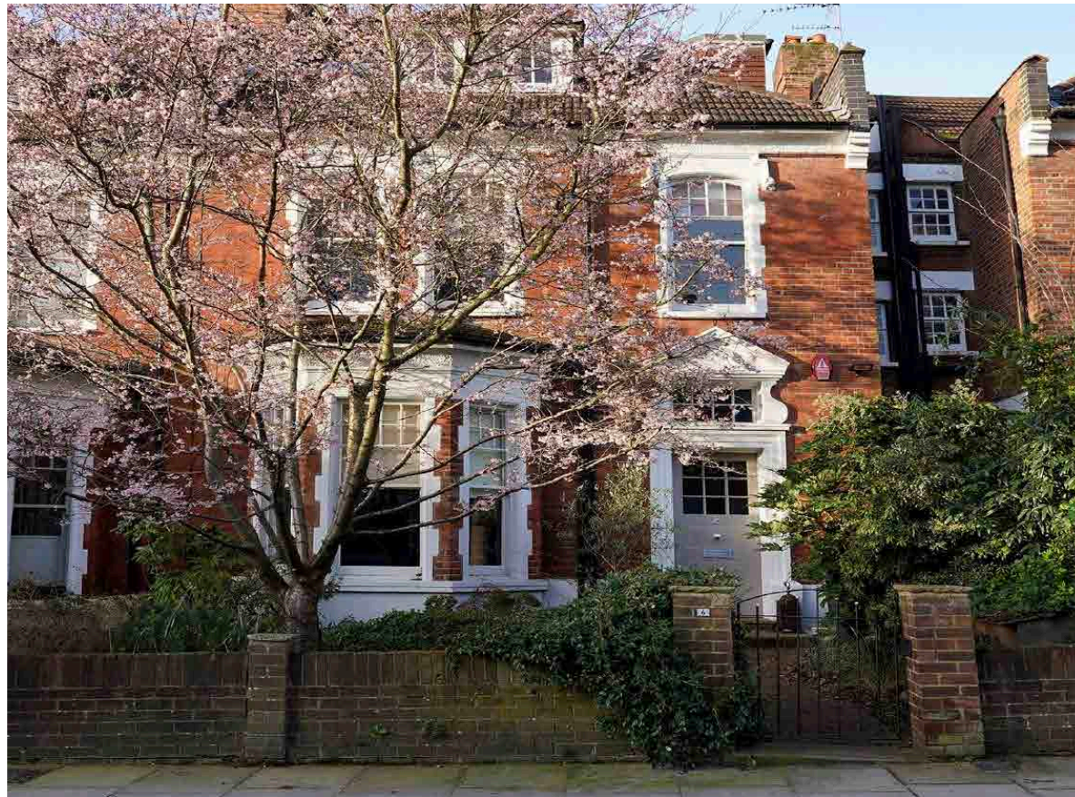
6 Clifton Road - View from street
