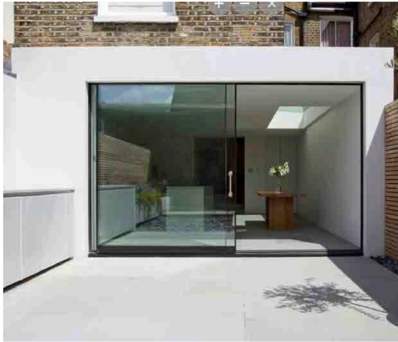
White render facade to extension
