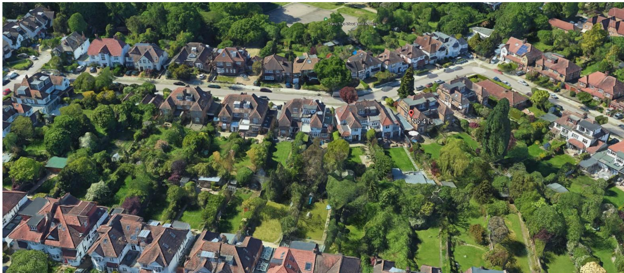
Rear elevations of 12–34 Fordington Road (even numbers)
