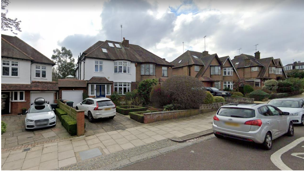
View of the property from Fordington Road
