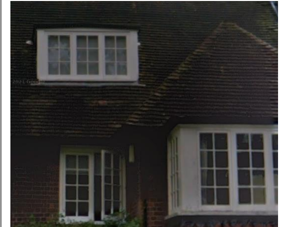
Figure 46 Overhanging eaves timber casement windows brickwork ridge tiles
