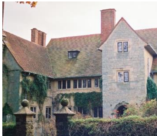
Figure 50 Little Thakeham – Entrance Front
