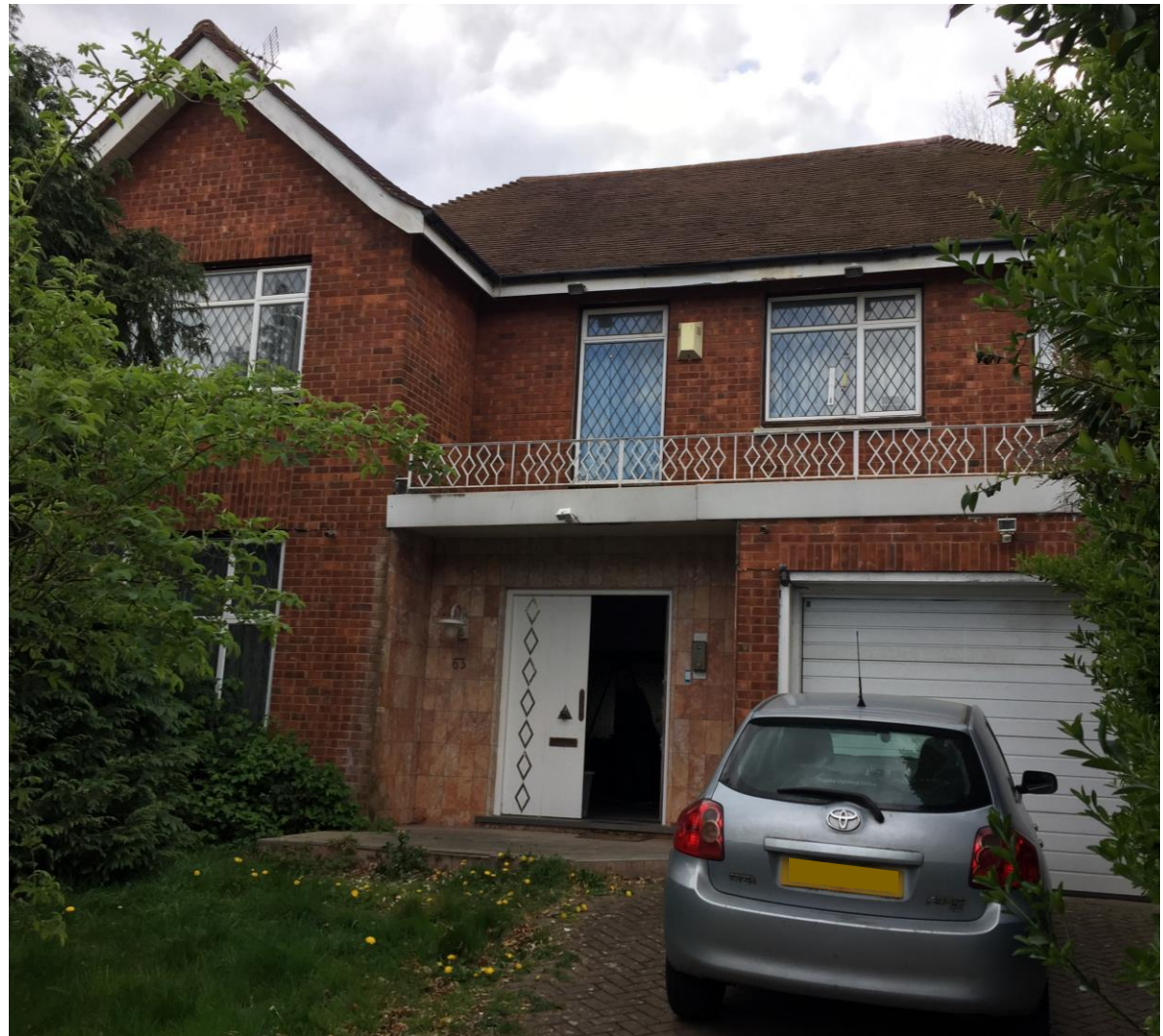
Figure 2 – View of front of property
