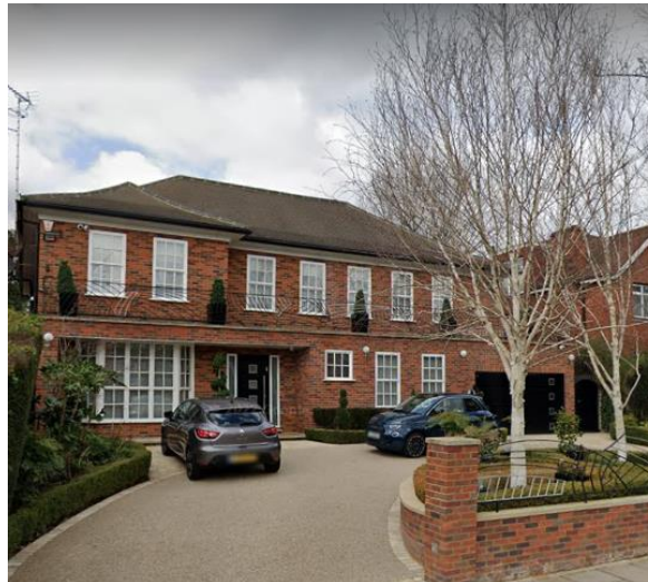
Figure 43 View of No 63 Sheldon Avenue
