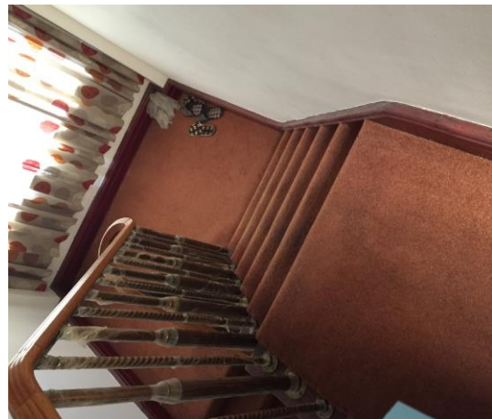
Figure 20 View of stairs
