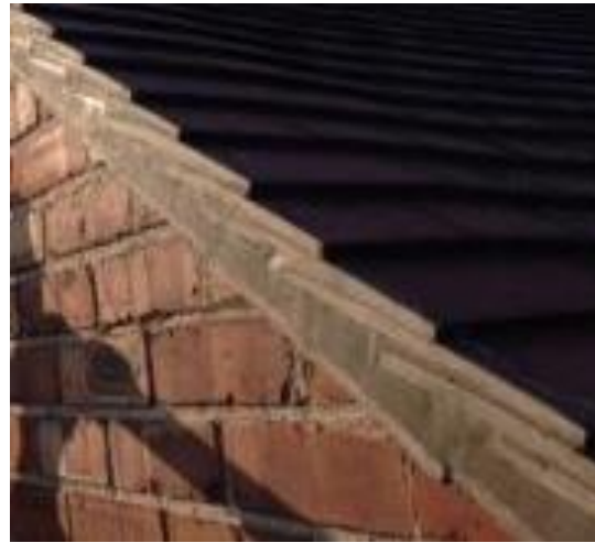
Figure 66 Exposed edge of plain tile bedded in mortar – wet verge detail
