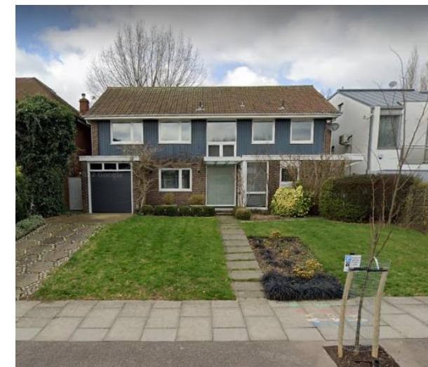
Figure 44 View of No 65 Sheldon Avenue
