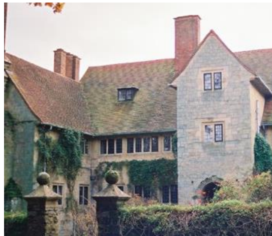
Figure 50 Little Thakeham – Entrance Front
