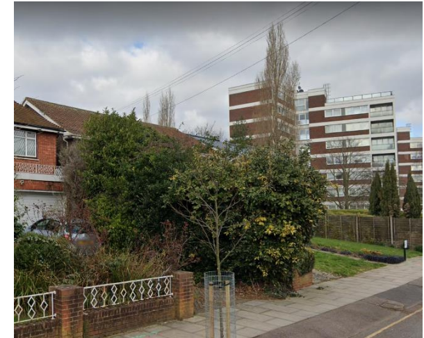
Figure 42 View of Tower block in setting of site
