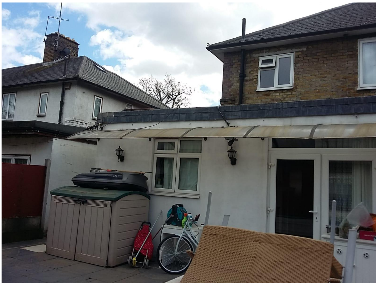
Pic.4 Rear Elevation Nos.11 & 13
