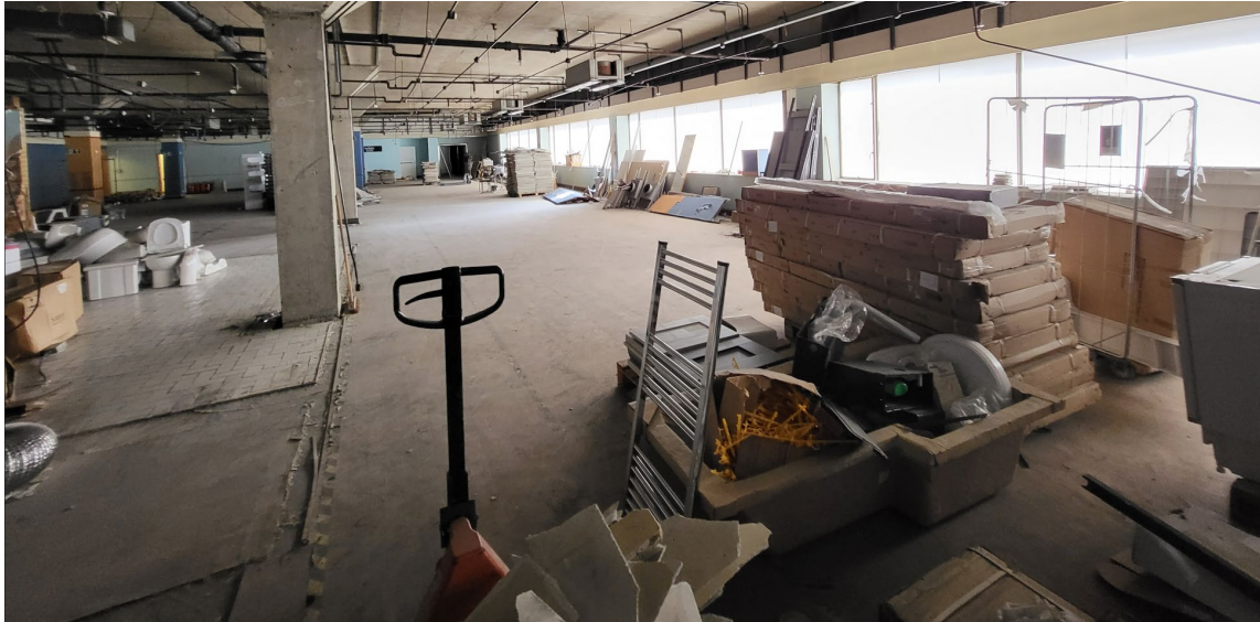
Above: Existing first floor used as a storage facility
