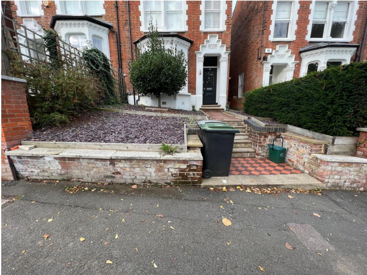
THE EXISTING FRONT BOUNDARY WALL TO 32 CROMWELL AVENUE
