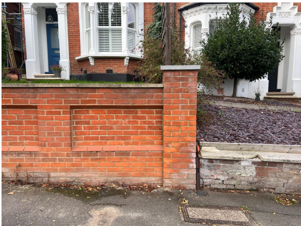
EXISTING NEW FRONT WALL AT 34 CROMWELL AVENUE ADJOINING THE APPLICATION SITE
