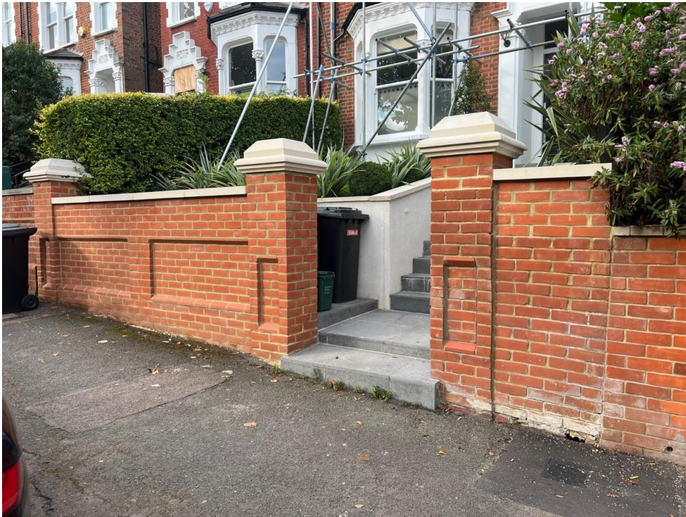
EXISTING NEW BRICK WALL AND BINS STORE AT 36 CROMWELL AVENUE
