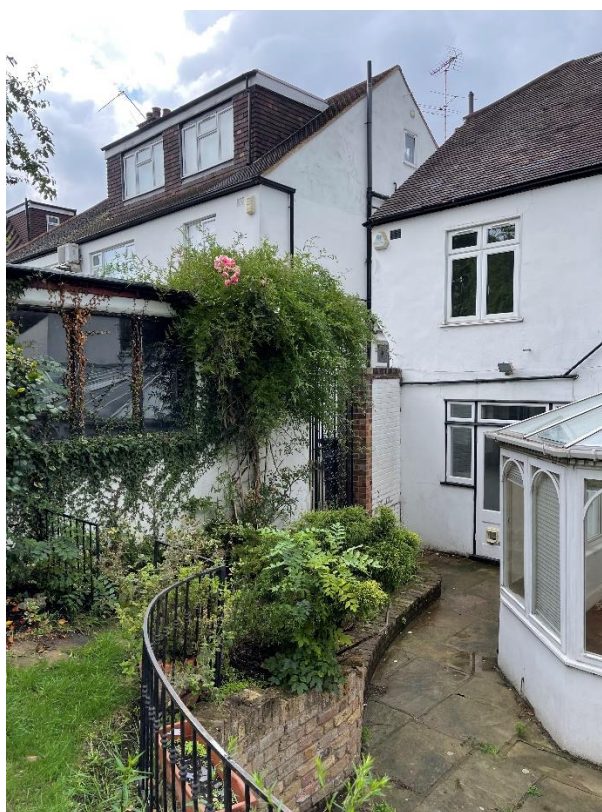
Change in level between between houses.
