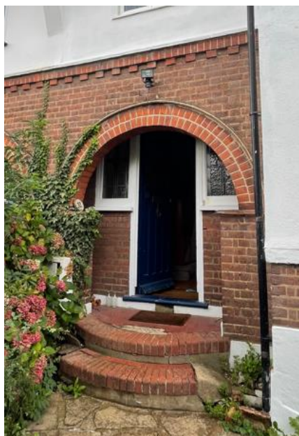
Front elevation and main entrance.
