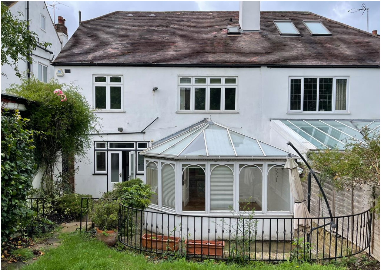
Applicant site, rear elevation, viewed from north east.
