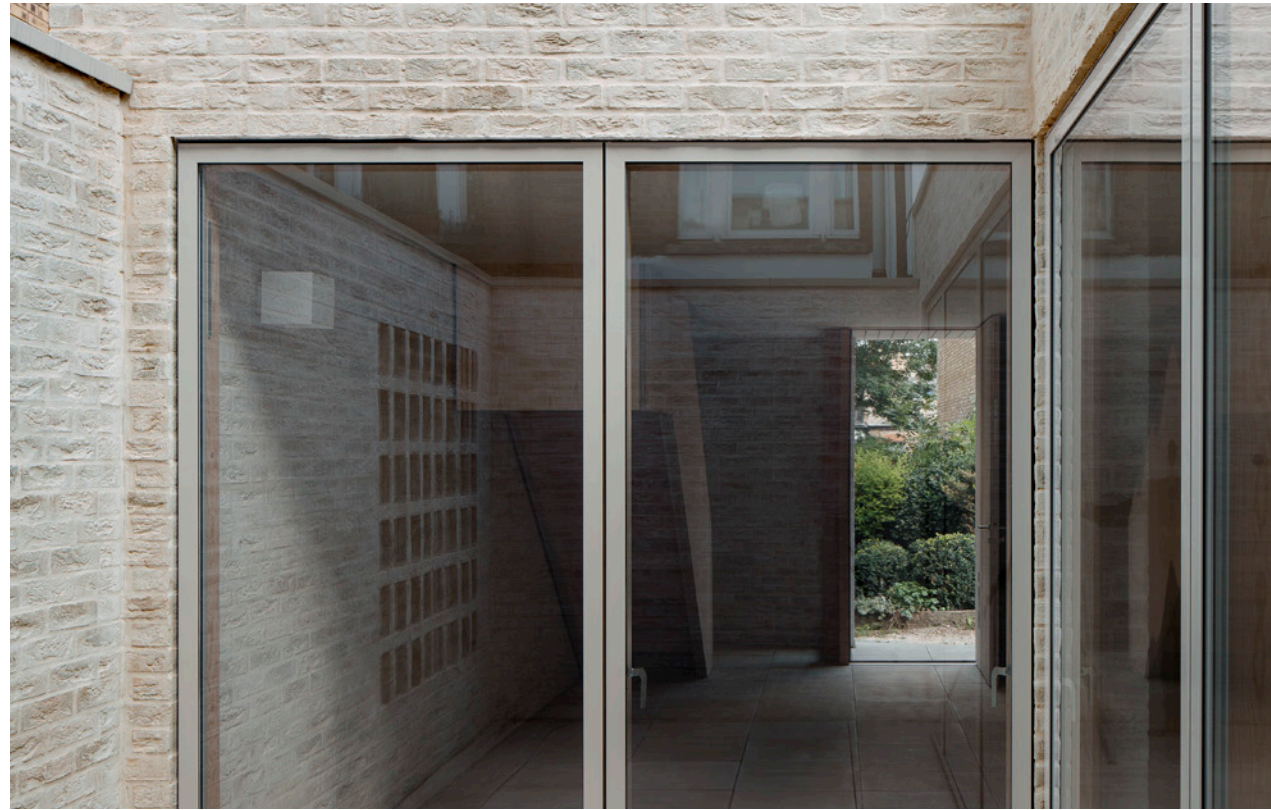
Light Buff coloured textured brickwork, flush white lime rich mortar. Powdercoated aluminium fenestration with internal timber framing.
