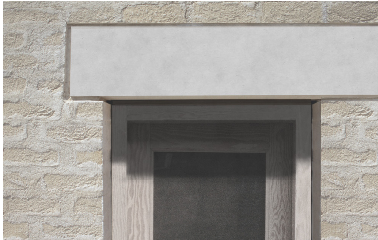
Timber entrance door. Pale colour precast concrete lintels. Light Buff coloured textured brickwork with flush white lime rich mortar.
