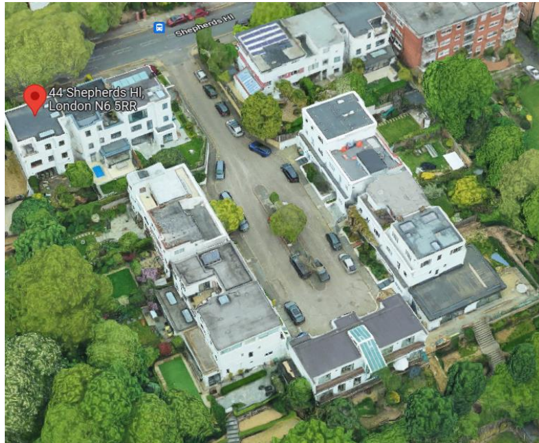
Figure 5: image showing glazing at roof level of surrounding properties.
