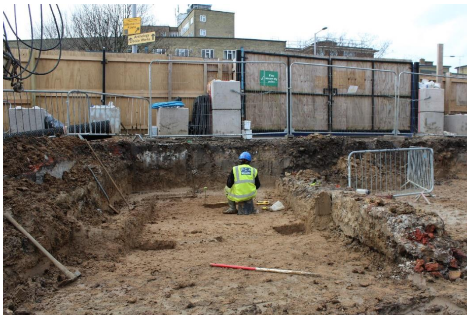
Plate 6: Working shot looking west (1m scale)
