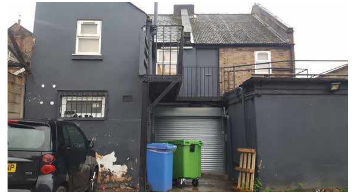
View of the rear of the property (north of Site).
