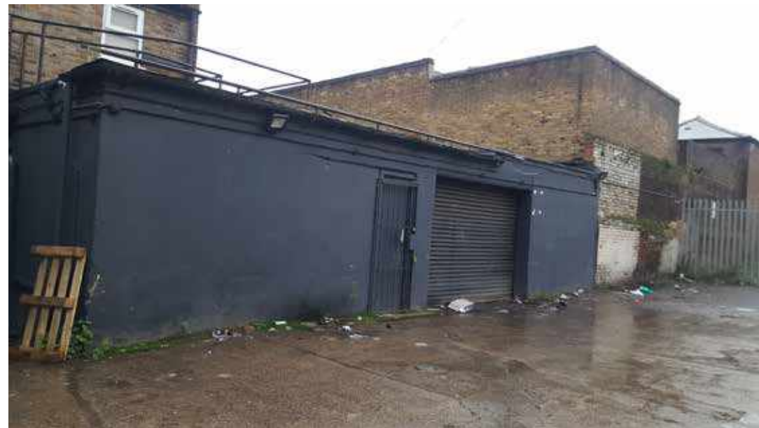
View of the storage area situated in the rear of the property from Percival Court.
