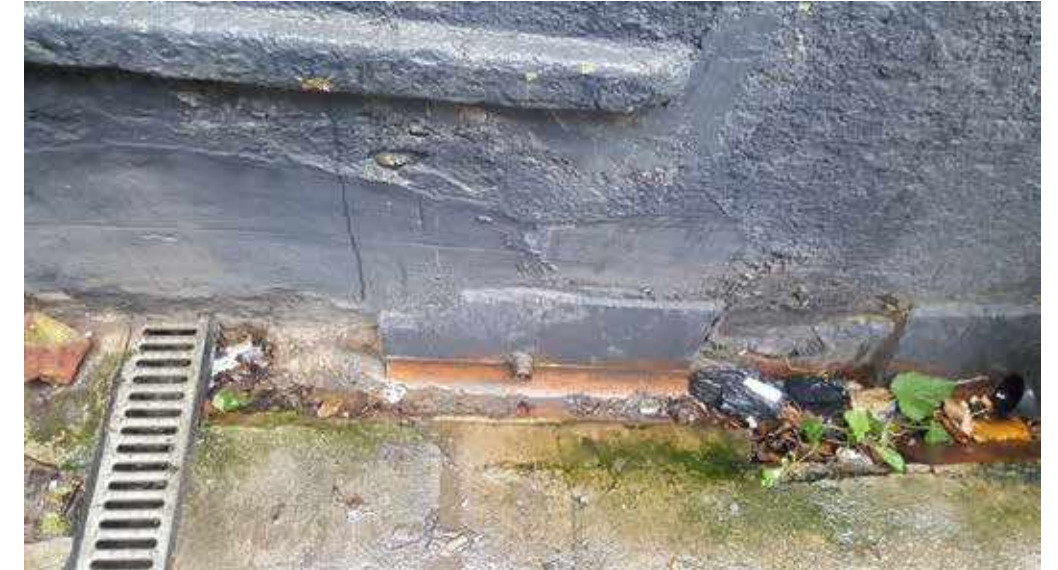
Drainage inset around the rear of the property (north of Site).
