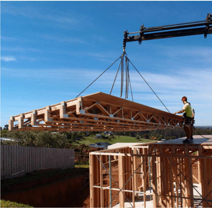
40 Pre-fabricated floor cassette being craned into place
