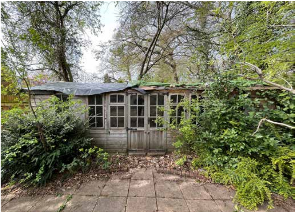
12 Existing Rear Garden Shed
