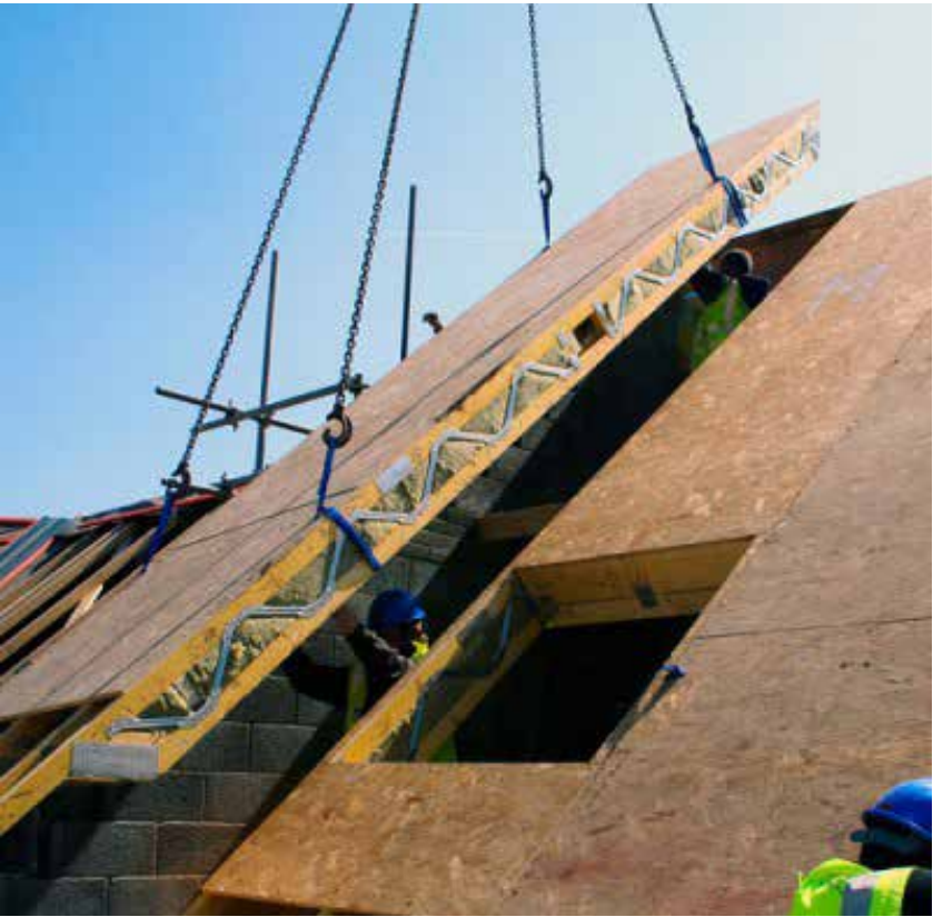
39 Pre-fabricated roof cassette being craned into place
