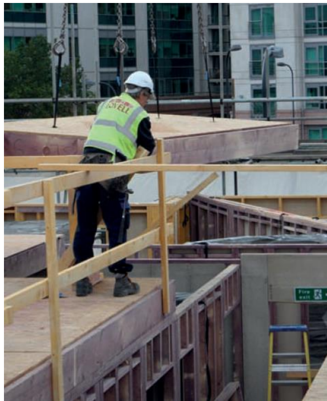
Figure 4 - Floor Panel being lowered
